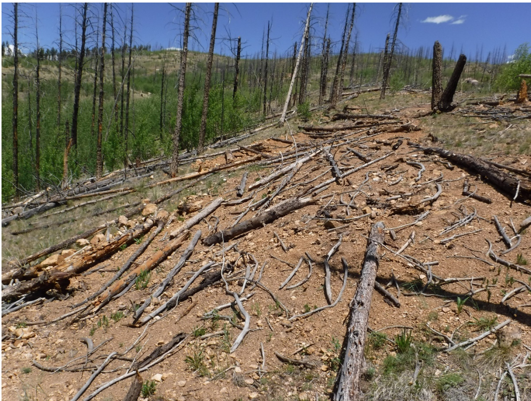
Photo 6. Backfilled excavation, small trees used to control erosion and aid revegetation efforts; looking north.
