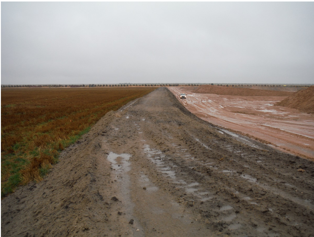
Photo 6. Active overburden face and product stockpiles, mine advancing to the west (left); looking north.
