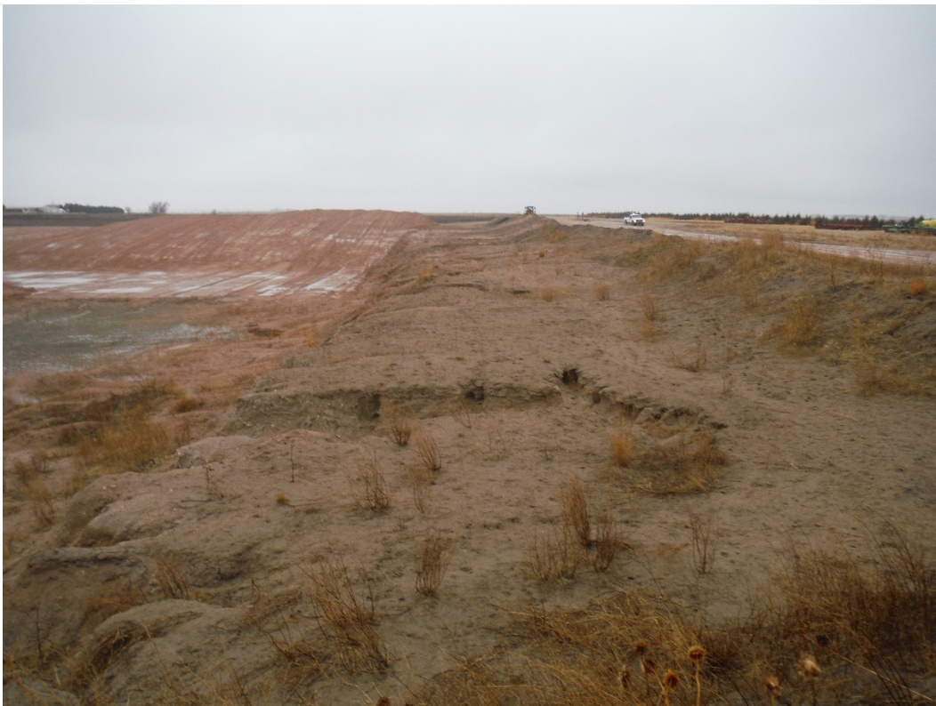
Photo 2. Northern pit slope; looking west.
