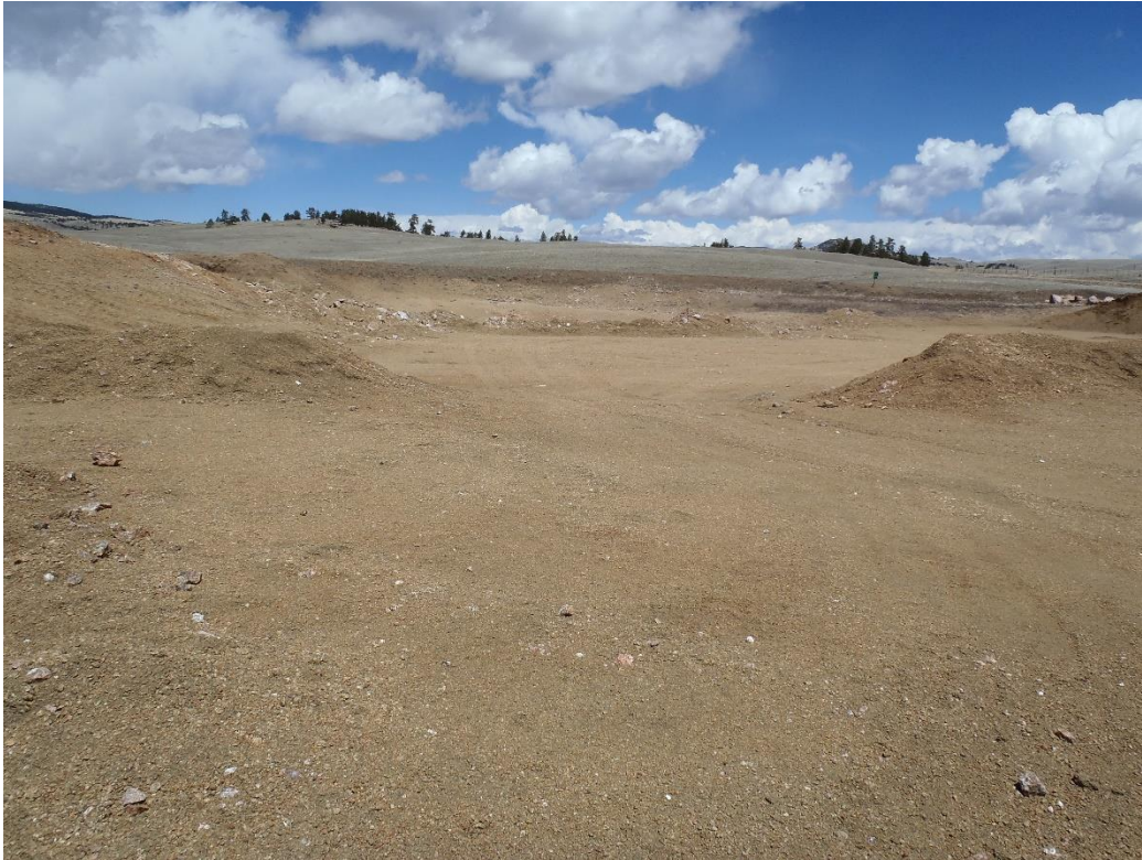
Photo 4. Highwalls, on average ~10 feet in height appeared stable (looking NNE).
