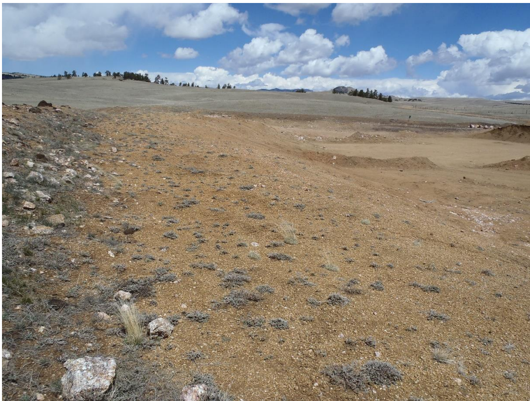
Photo 1. Highwalls appeared to be near 3H:1V (looking NNE).
