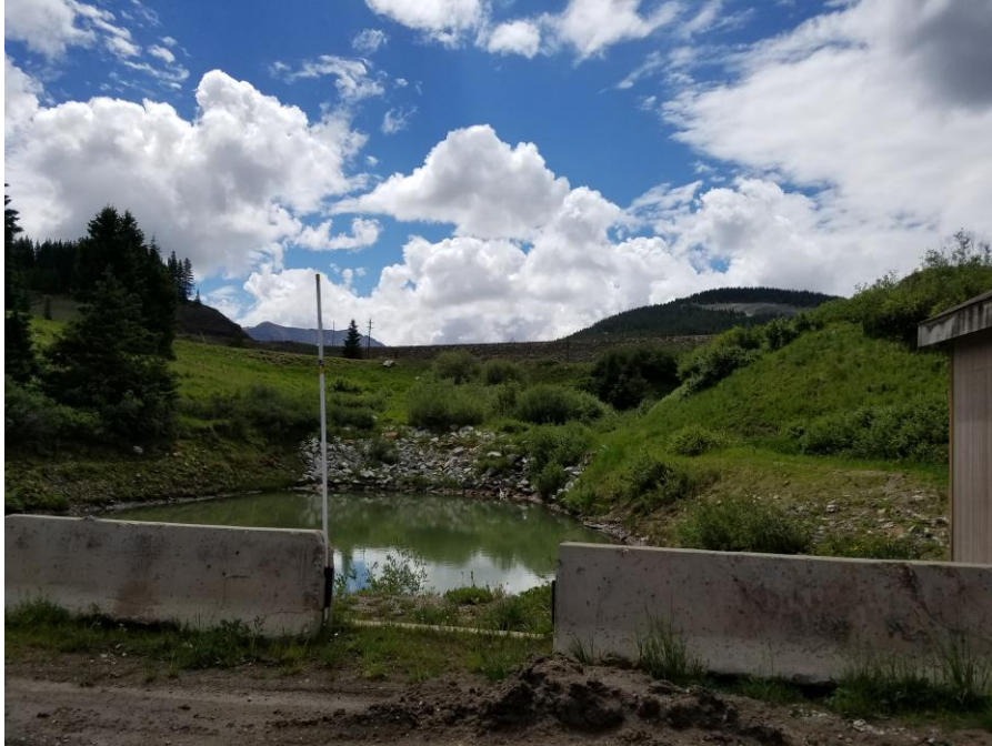
Figure 5. Robinson Lake Seepage and Cut-off Wall.
