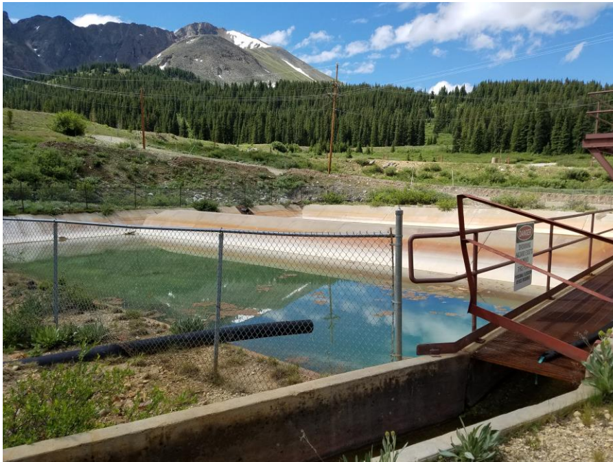
Figure 2. Decant ponds at Storke Wastewater Pump Station.
