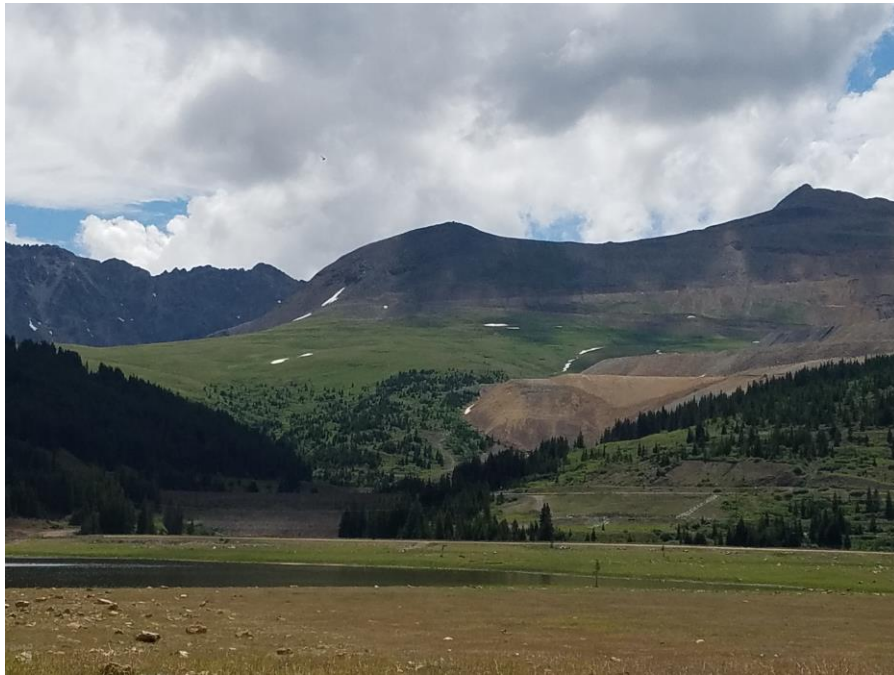
Figure 4. From the south end of the Robinson TSF looking east toward the OSFs.
