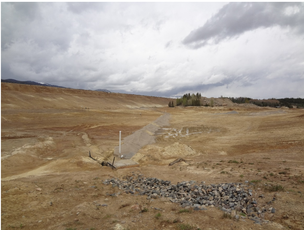
View of French drain on the southern portion of the 3-Dam stepback bench
