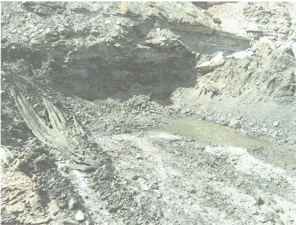
Pic. 2 –Under drain exposed at base (south end) of the embankment/waste pile .
