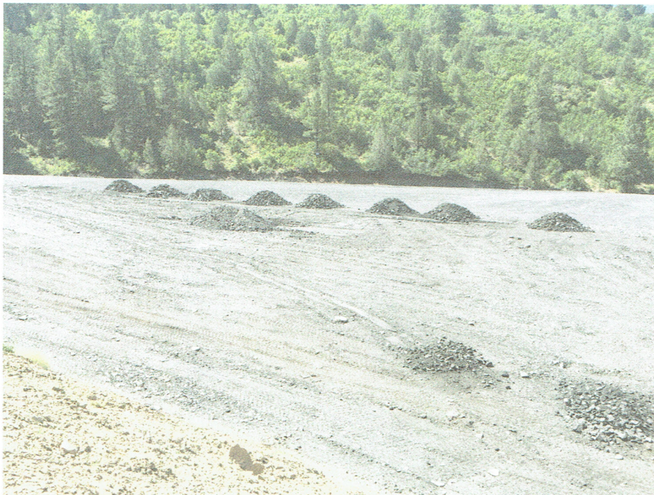
Pic. 4 – Embankment material ready for placement at top of embankment.
