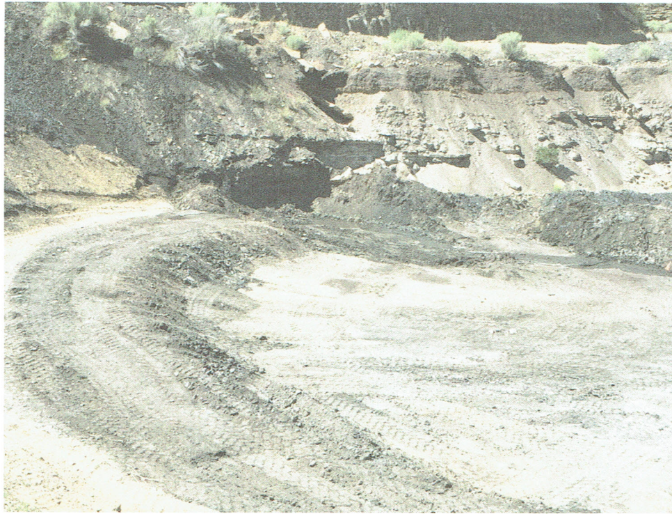
Pic. 3 –Exposed under drain, existing ditch located to west at base of natural embankment.
