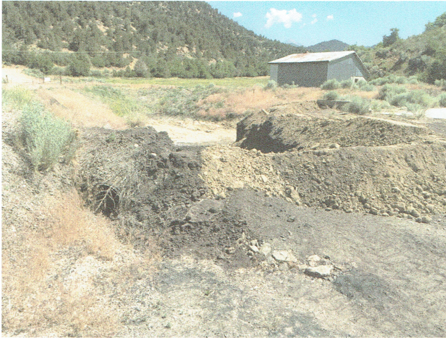
Pic. 3 – Pipe inlet, east pond, temporary embankment material placed.
