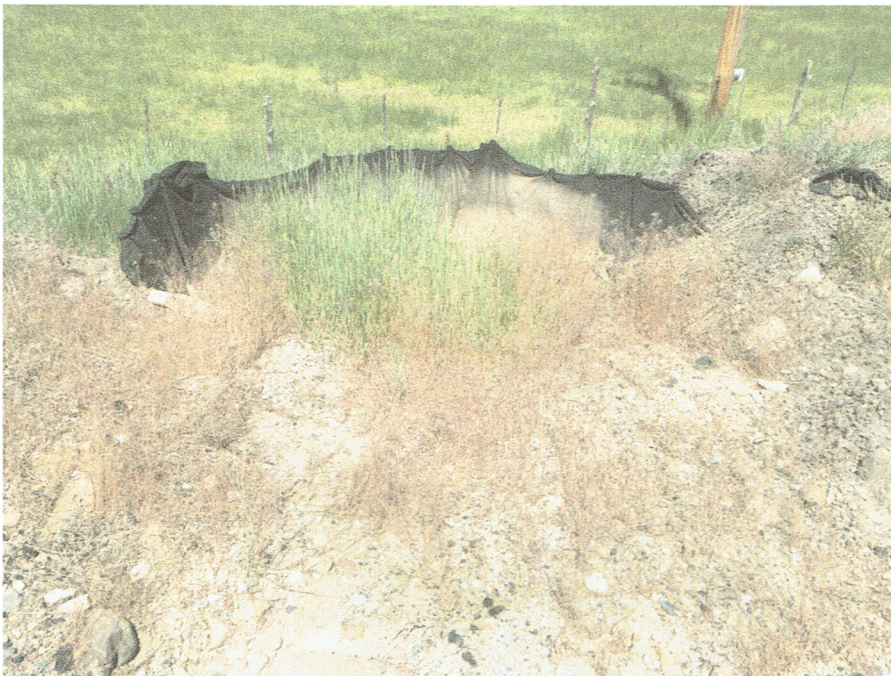
Pic. 4 – Sediment traps along west side of driveway in good condition.
