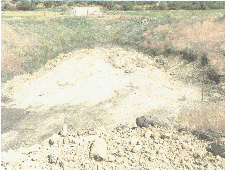
Pic. 1 – East pond, fill material installed in base.
