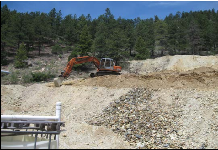
1. Excavator removing material from within tailings impoundment.
