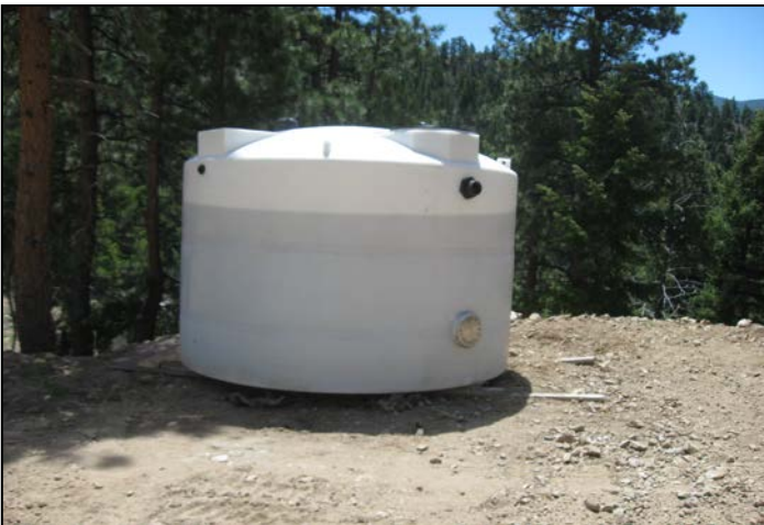
3. Tank used for the interim storage of liquid pumped from tailings impoundment.
