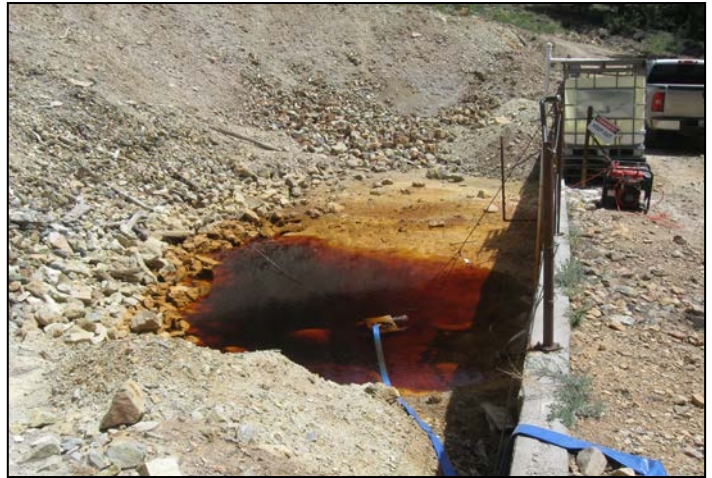
2. Residual liquid within tailings impoundment.
