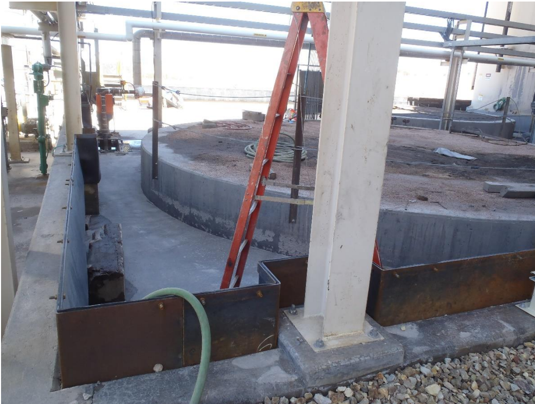
Photo 1. Completed vat leach tank secondary containment construction (steel plate & rubber membrane).
