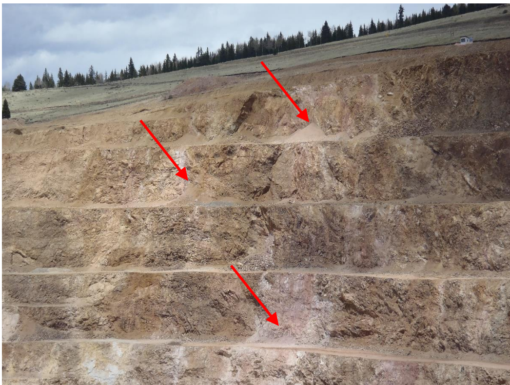
Photo 12. WHEX highwall – minor sloughing (looking NE).
