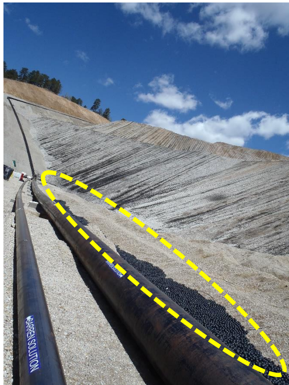
Photo 6. Bird balls in the stormwater collection trench northeast of ADR2 (looking NE).
