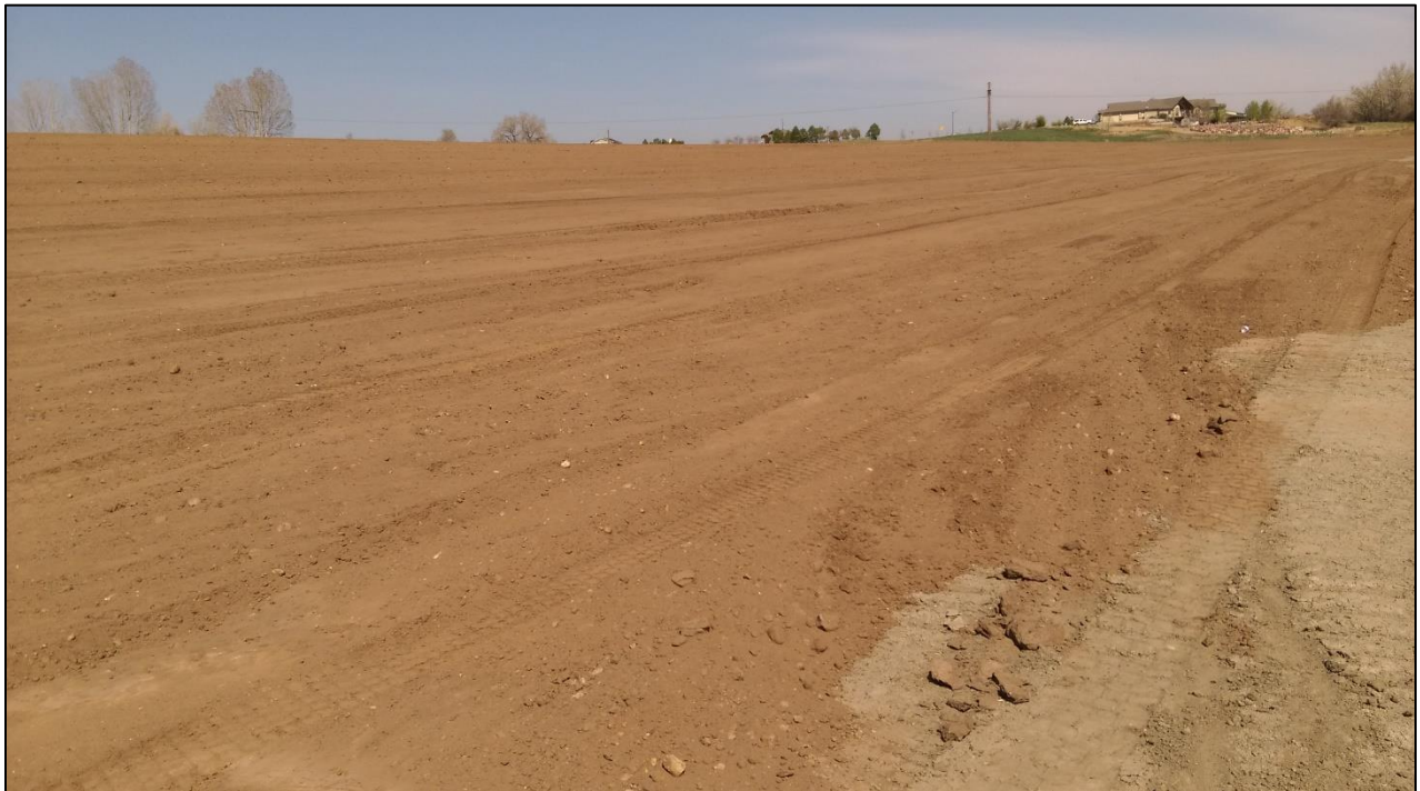
Photo 12. View looking north across western bank of West reservoir recently graded to flatter than 3H:1V, retopsoiled and seeded.
