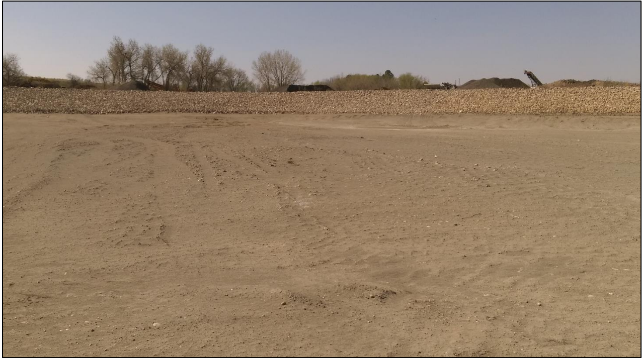
Photo 3. View looking southwest from floor of East reservoir, showing riprap placed along southwestern bank of reservoir.
