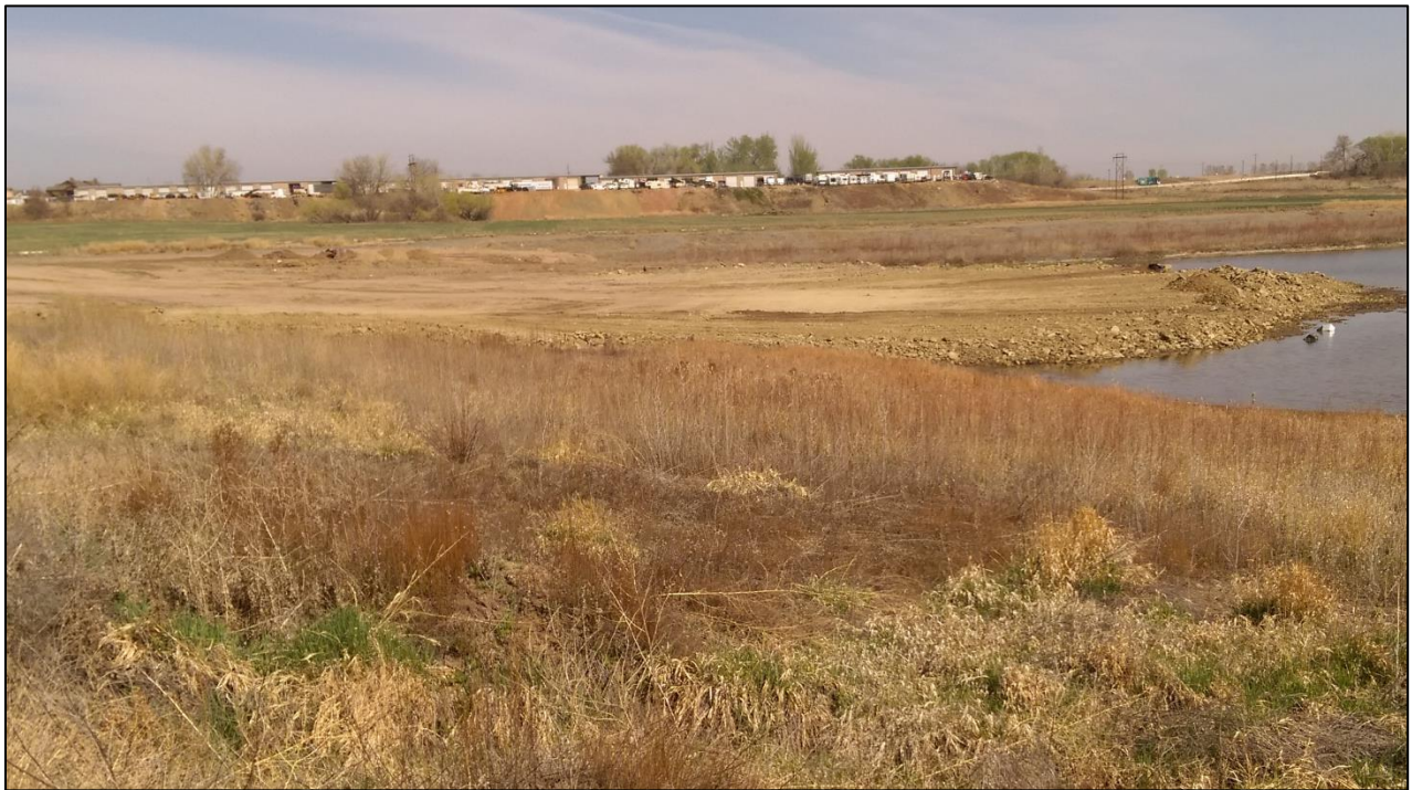
Photo 8. View looking northeast across backfilled northwestern portion of pit shown in Photo 7.
