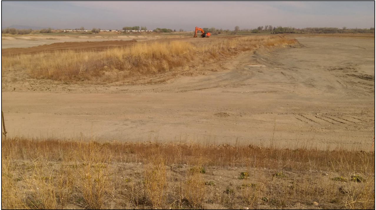
Photo 5. View looking north from southern bank of East reservoir, showing large topsoil stockpile stored on floor of reservoir.
