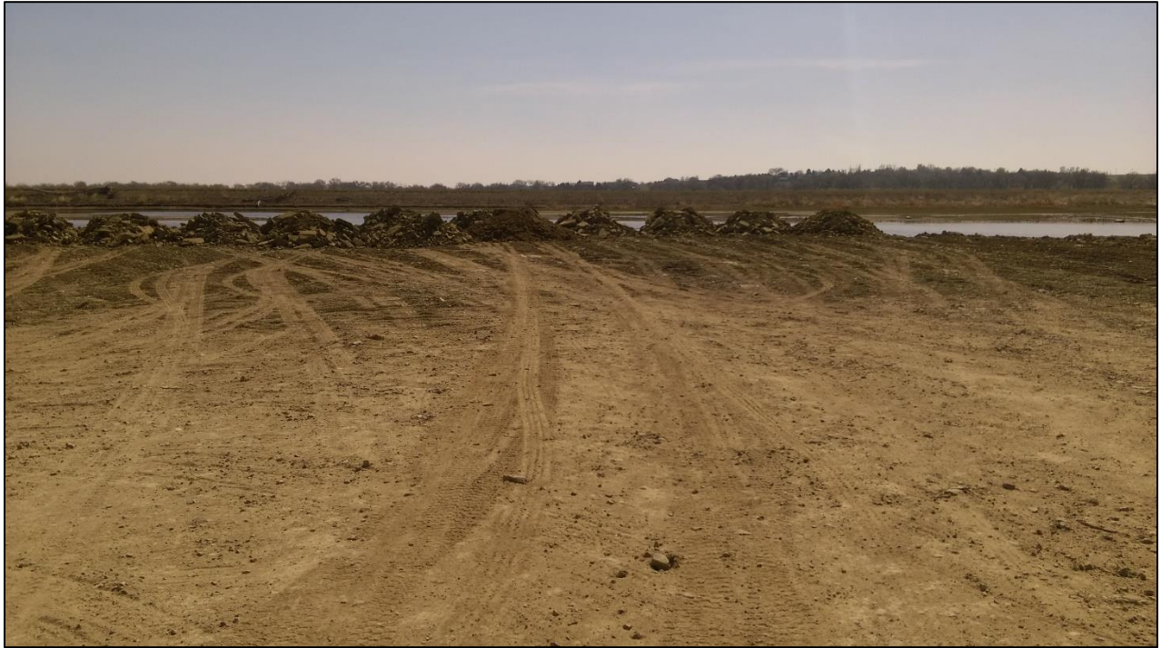
Photo 9. View looking southeast across backfilled northwestern portion of pit shown in Photo 7.
