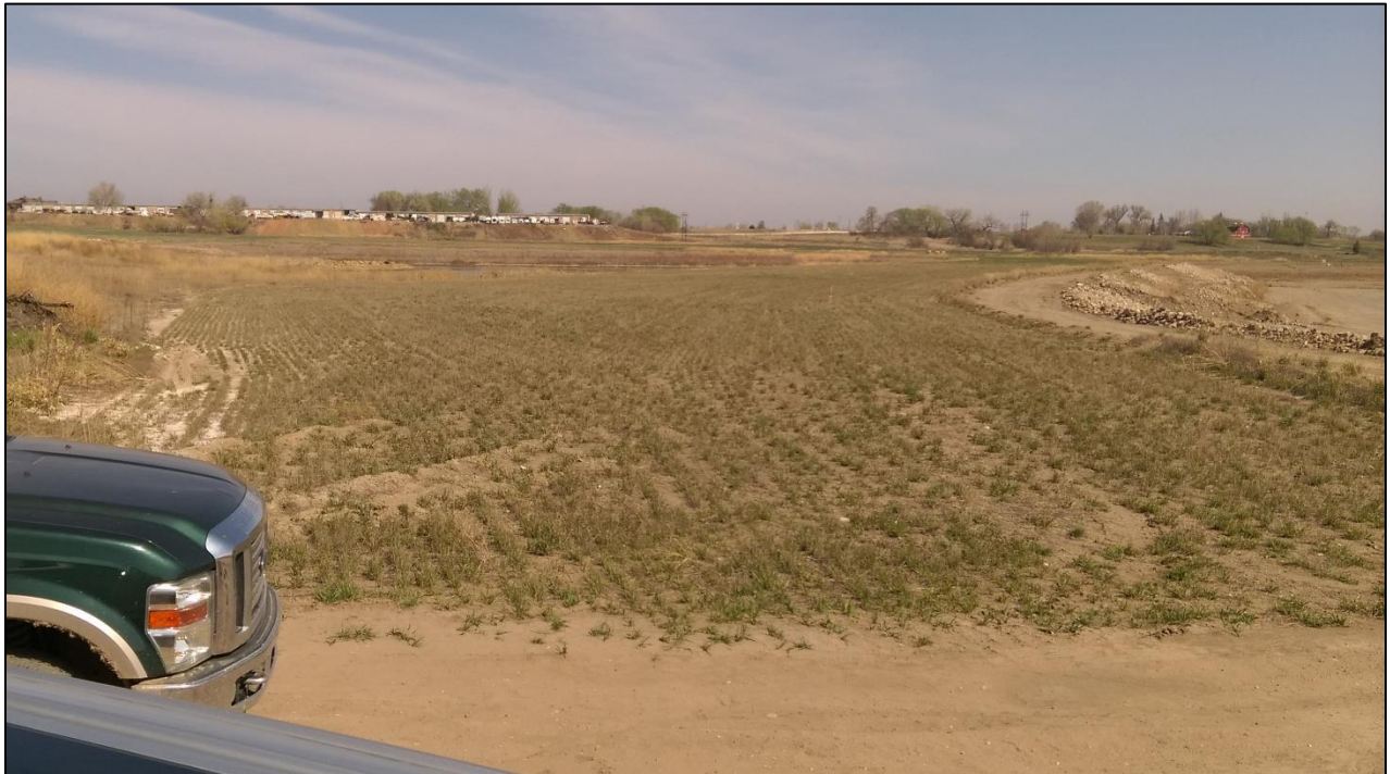
Photo 14. View looking north across roadway embankment constructed along City of Loveland right-of-way. Note roadway is stable with good grass cover. Haul road in foreground is reservoir access road.
