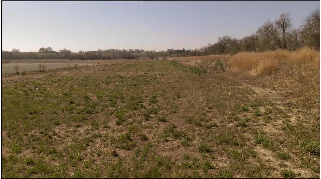
Photo 13. View looking south across roadway embankment constructed along City of Loveland right-of-way. Note roadway is stable with good grass cover. City of Loveland will complete final construction of road after permit is released.
