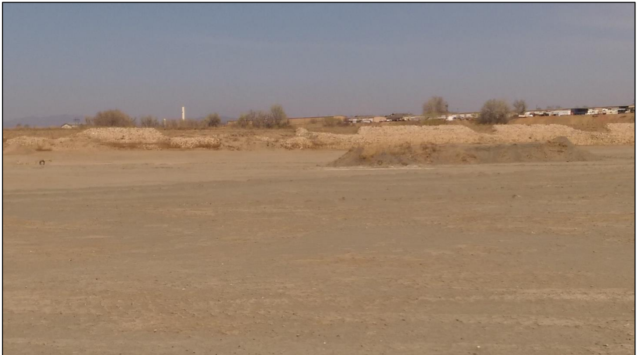
Photo 4. View looking northwest from floor of East reservoir, showing riprap placement along western bank in progress.
