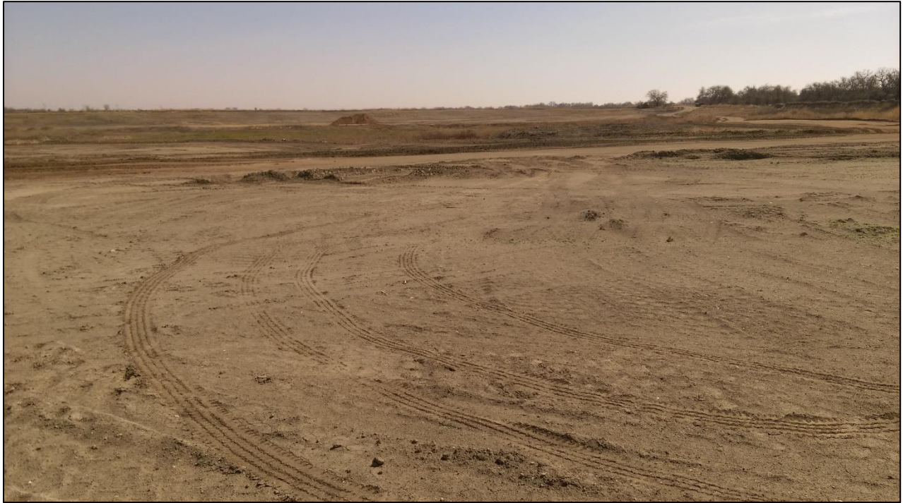
Photo 11. View looking east from floor of West reservoir. Note reservoir is dry.
