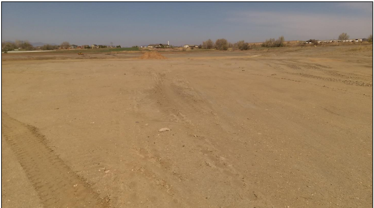
Photo 10. View looking north from floor of West reservoir. Note reservoir is dry.
