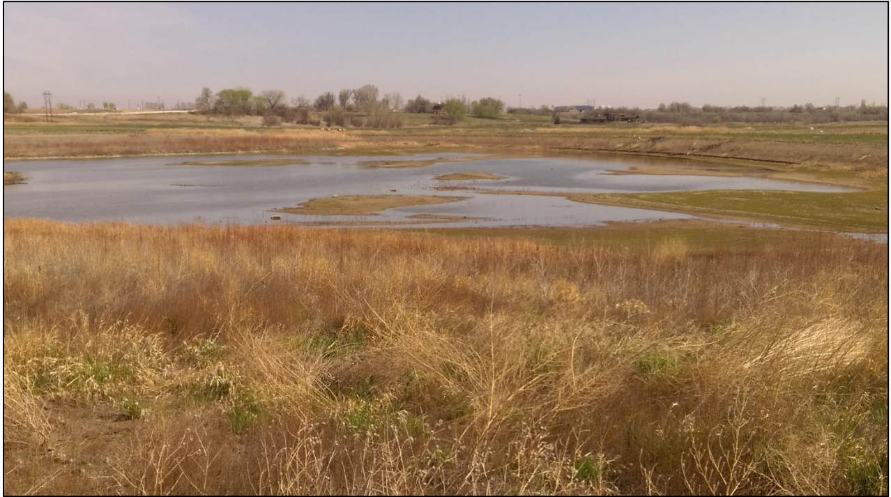
Photo 7. View looking east across northwestern portion of East reservoir separated by roadway embankment constructed along City of Loveland right-of-way. Note water present in pit during inspection.
