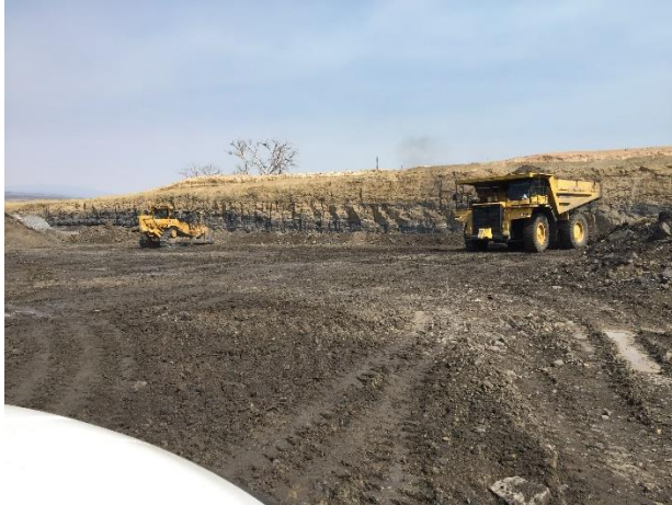
Photo 1 – Backfilling Main Pit
