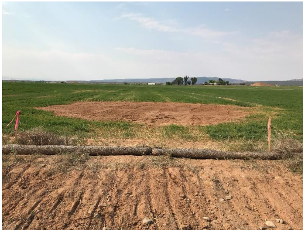
Photo 7 – Topsoil Depression Repair
