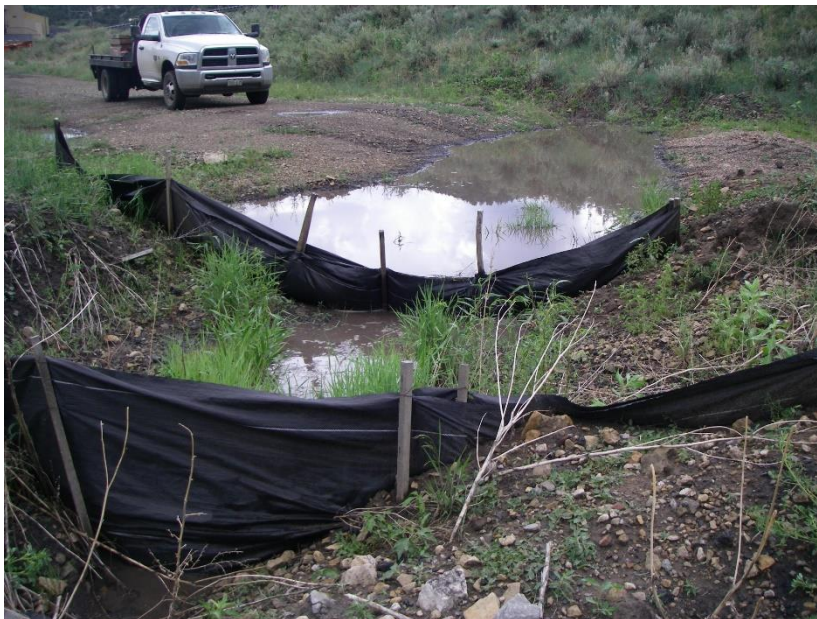
Silt fence below SAE beside Pond 007A
