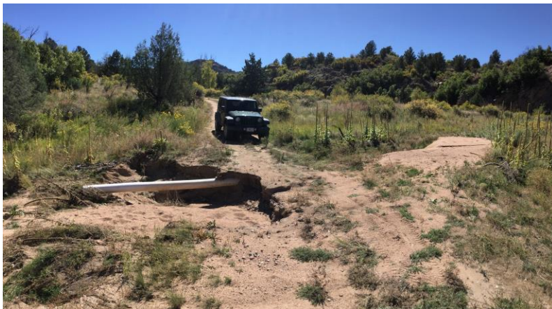
Photo 2: Erosion along the access road further east of the locked gate on private land (on the way to the site). Note the pre-existing PVC pipe which the private landowner might have installed to decrease overland flow.
