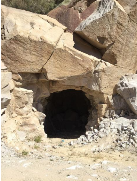
Photo 7: The inactive highwall on the west of the site, where rain water pools prior to flowing into the hole going through the access road.
