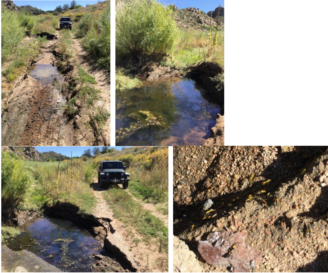
Photo 2: Erosion along the access road further east of the locked gate on private land (on the way to the site). Note the pre-existing PVC pipe which the private landowner might have installed to decrease overland flow.
