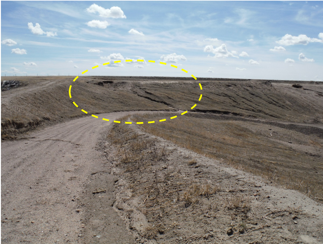
Photo 3. Erosional feature of concern; looking south.
