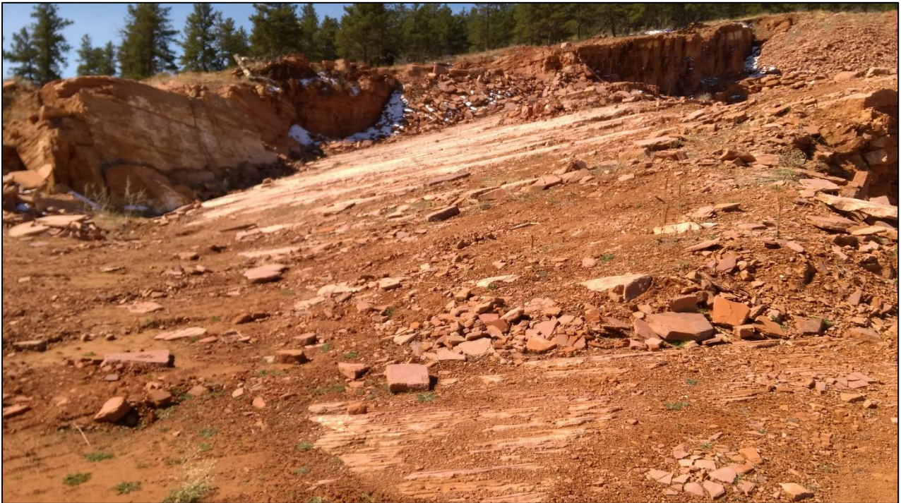
Photo 1. View looking southwest at eastern portion of highwall present along southern edge of site.
