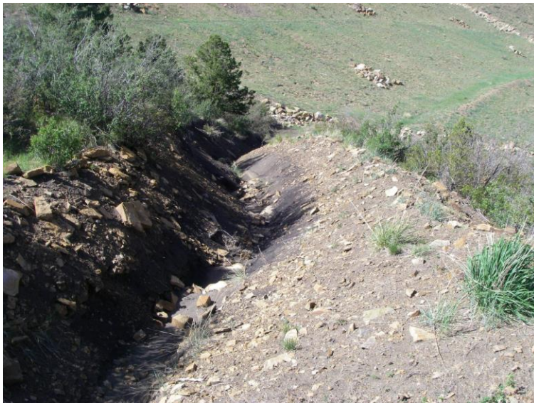
Contour ditch on small portion of Fill 7
