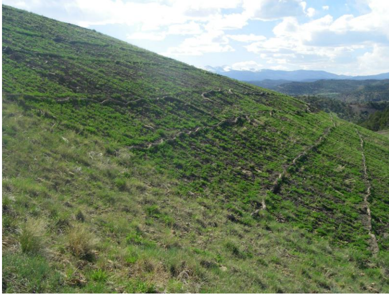
Need for wattle repair on hill west of the shrub plot (above dump area for pond cleanings)
