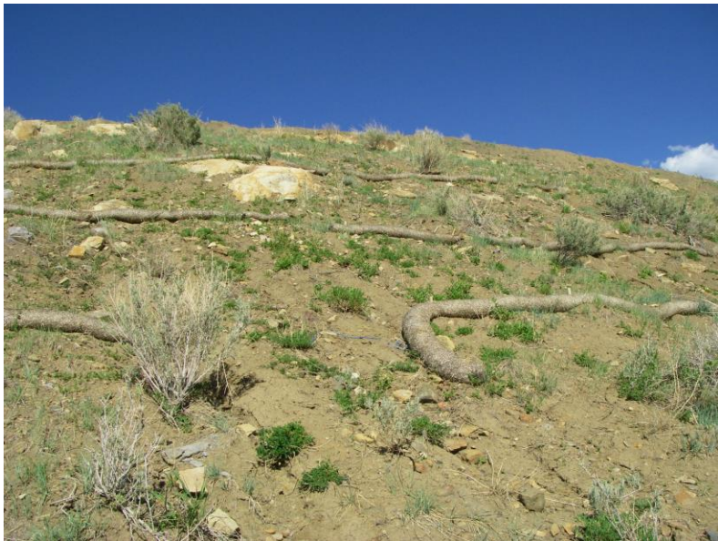
Need for wattle repair on west side of “the knob”
