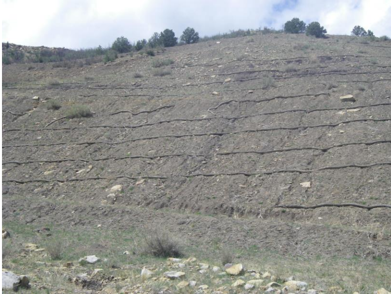
Damaged wattles on hill above Pond 6
