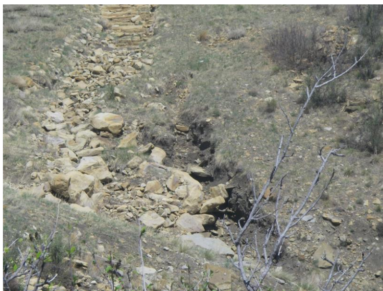
East channel of Fill 9 – possible need for more riprap
