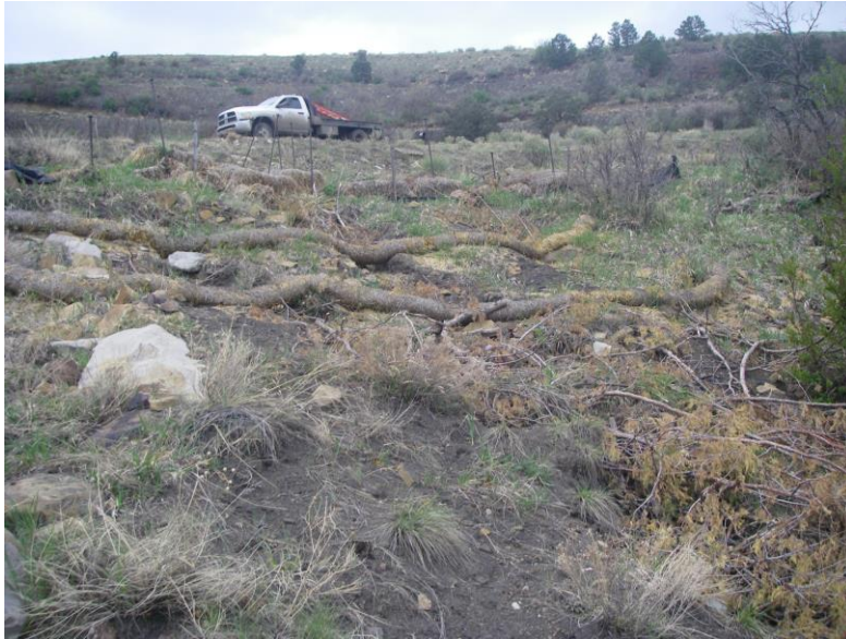
Sediment and erosion controls below Pond 9
