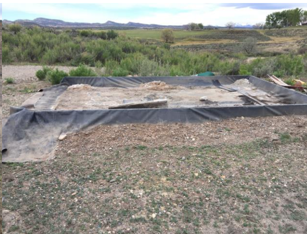
Photo 4 – Pond NH1 Pump Station
