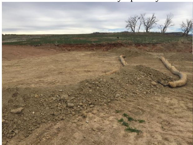
Photo 5 – End of Pond 002 North Ditch
