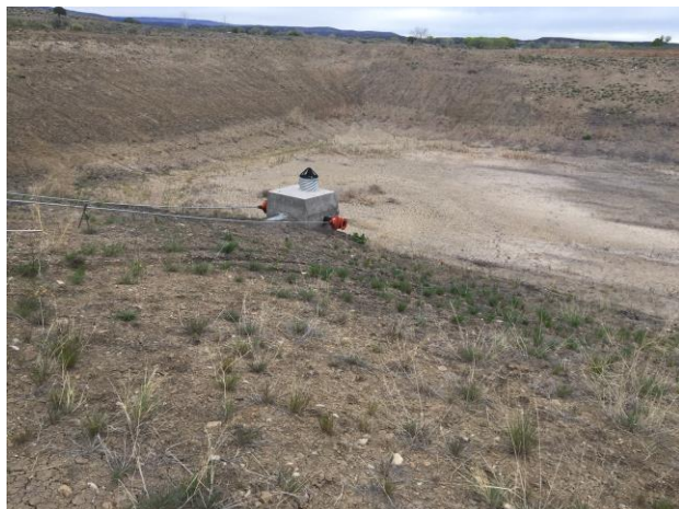
Photo 3 – Pond 002 – Primary Spillway
