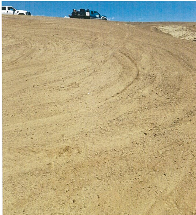
Picture 3: Seed and soil pockets covered by drag pulled by ATV
