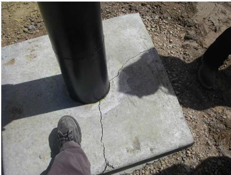
Cracked base at MW-4
