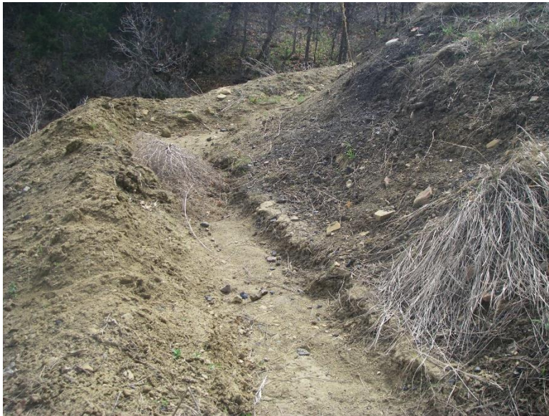
Ditch at plant growth medium storage area near Refuse Pile Recently cleaned but needs more maintenance
