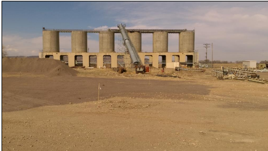
Photo 2. View looking north, showing six concrete load out silos present in central processing area.
