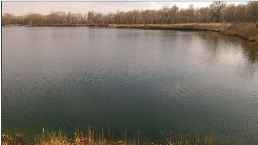
Photo 8. View looking southeast across Lake 1 from western shoreline. Lake shorelines are graded to 3H:1V or flatter with established vegetation.
