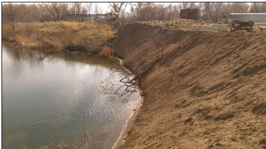
Photo 9. View of portion of western shoreline of Lake 1, showing slopes of approximately 1.5H:1V.
