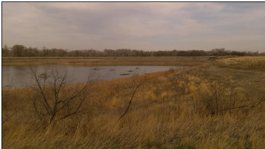
Photo 31. View of southern shoreline of Lake 4 graded to 3H:1V or flatter, stable with vegetative cover.
