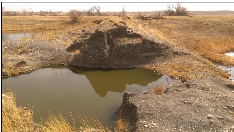
Photo 26. View of southeastern breached portion of berm and slurry wall liner around Lake 4. Lake 4 (at right) now connected to offsite lake (at left).
