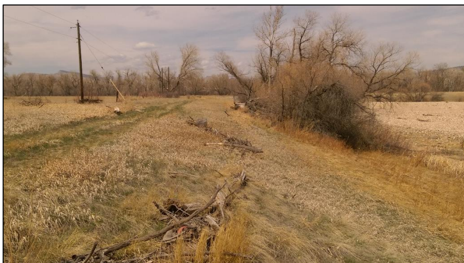
Photo 14. View of southwestern shoreline of Lake 2 graded to 3H:1V or flatter, stable with vegetative cover.
