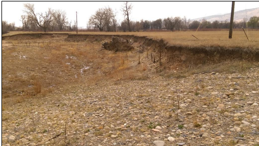
Photo 11. View of northwestern shoreline of Lake 2 damaged by September 2013 flooding. Bank slopes are steeper than approved 3H:1V gradient.
