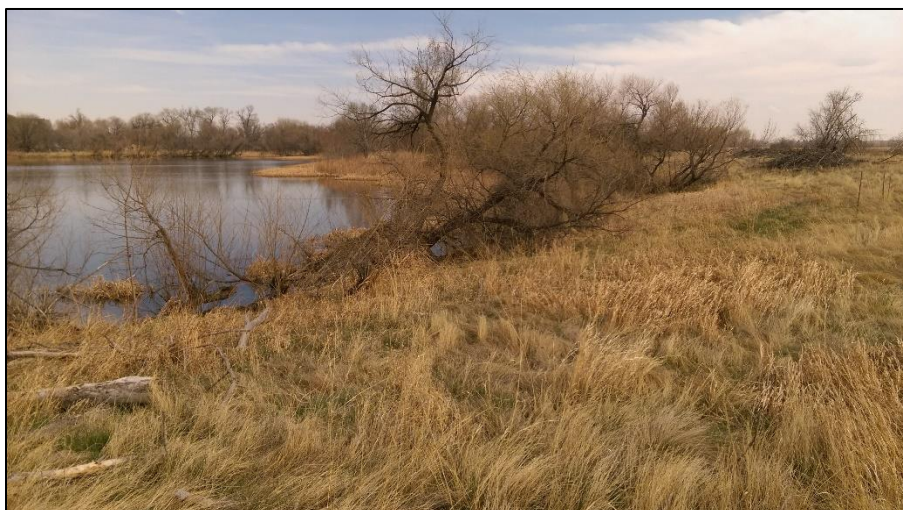
Photo 15. View of southern shoreline of Lake 2 graded to 3H:1V or flatter, stable with vegetative cover.
