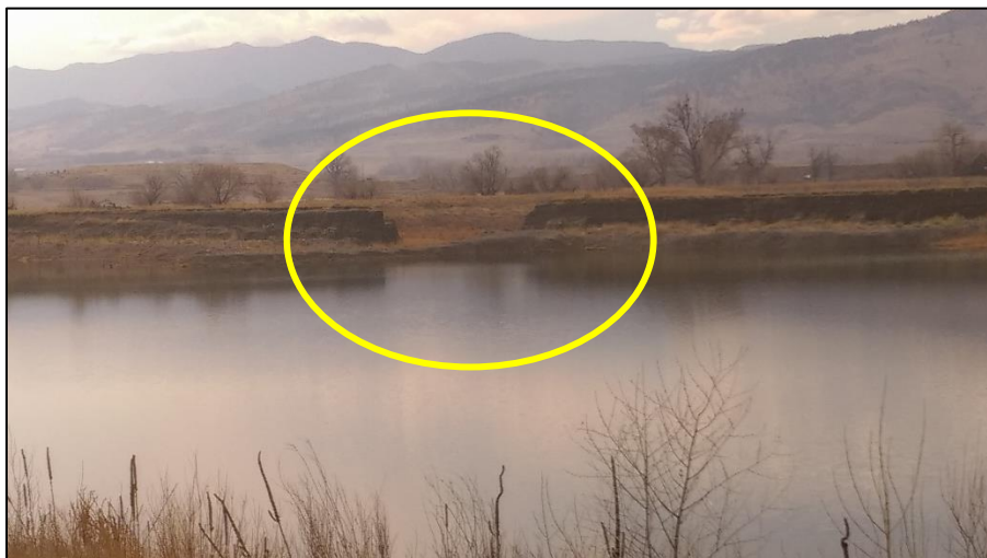
Photo 29. View looking west from eastern shoreline of offsite lake, showing breach in berm/slurry wall liner (circled) that had separated Lake 4 from the offsite lake.
