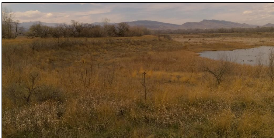
Photo 30. View of southern shoreline of Lake 4 graded to 3H:1V or flatter, stable with vegetative cover.
