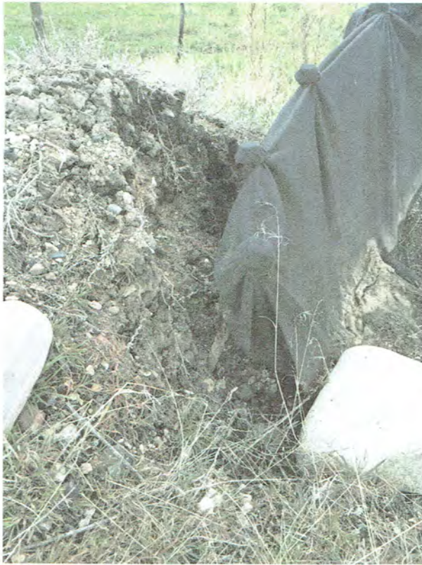
Pic. 3 – North sediment trap, west side of drive.
