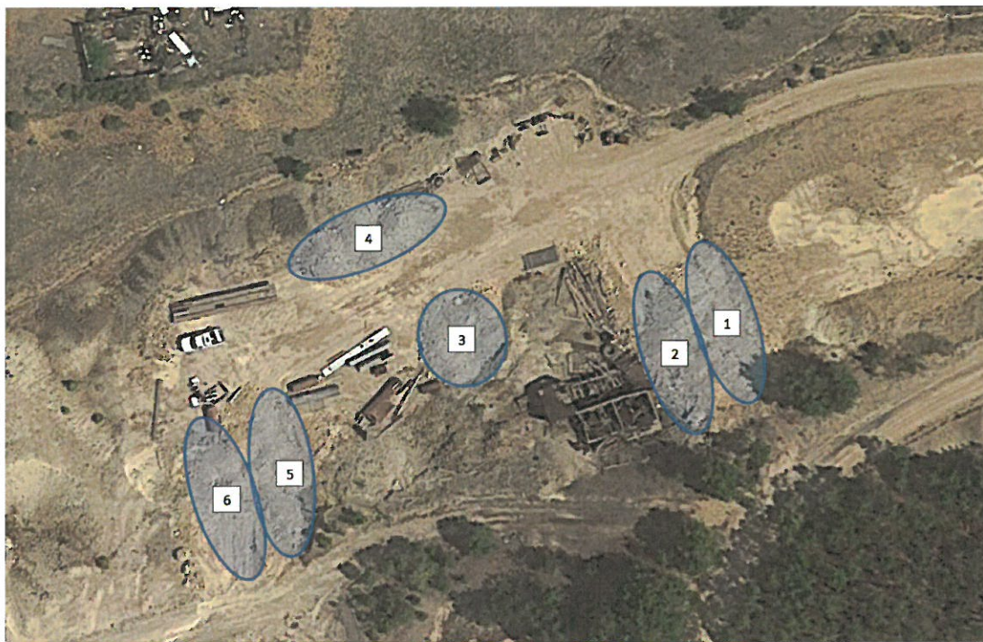
Figure 1: Plan view of the rock material piles immediately west of the Chicago Tunnel Mine.
