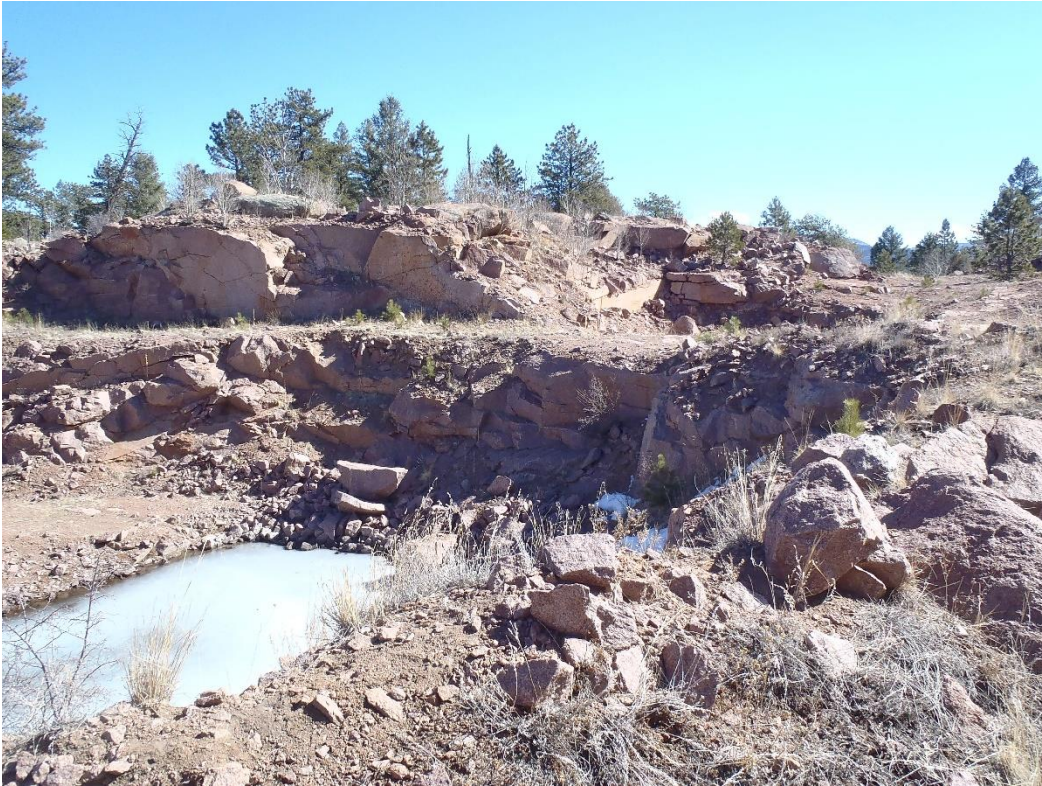
Photo 3. West pit highwall – note bench (looking east).
