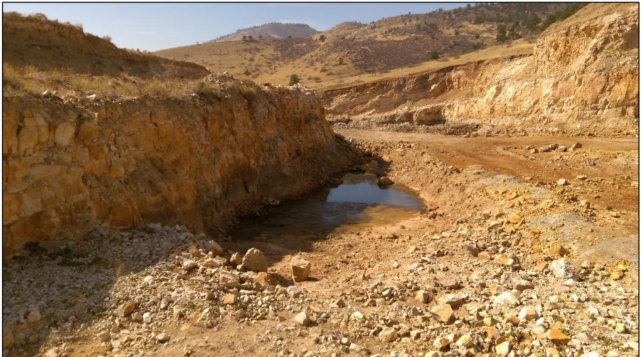
Photo 10. View looking south from northeastern edge of pit, showing small bermed sediment pond constructed along eastern edge of pit floor. Note very little water retained in pond.
