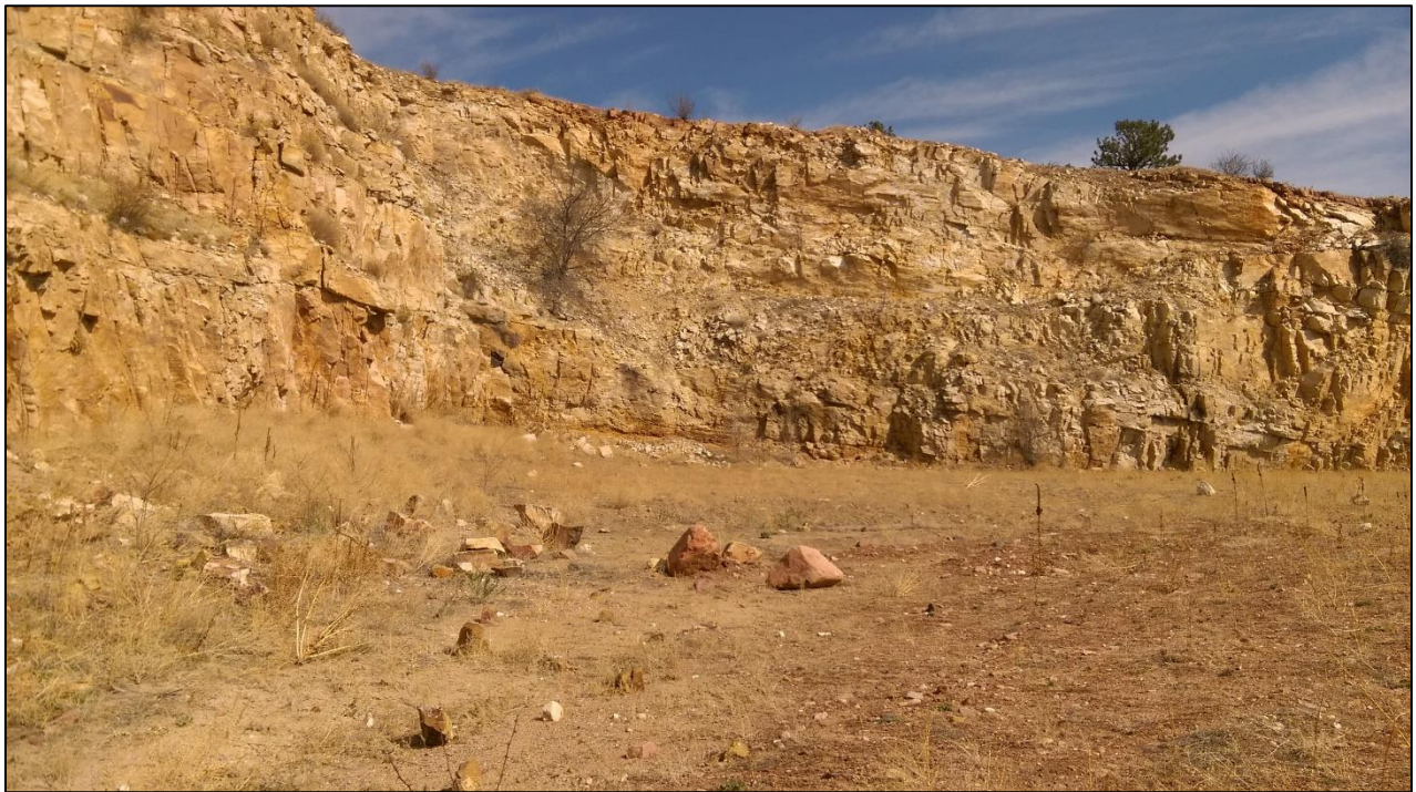
Photo 6. View looking north from pit floor, showing northern highwall. Note highwall bench slopes have gradients of approximately 0.5H:1V. Also note portion of pit floor (in foreground) that was backfilled and seeded in 2014.
