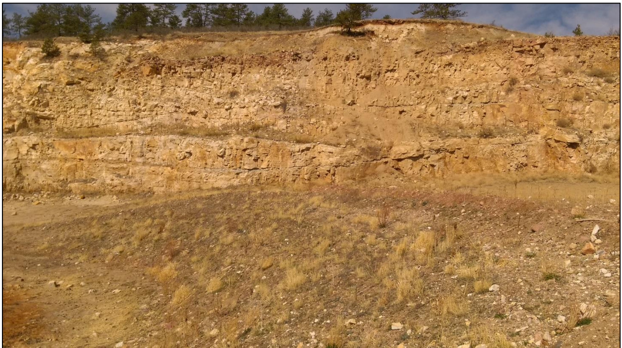
Photo 4. View looking west from pit floor, showing northern portion of western highwall. Note portion of pit floor (in foreground) that was backfilled and seeded in 2014.
