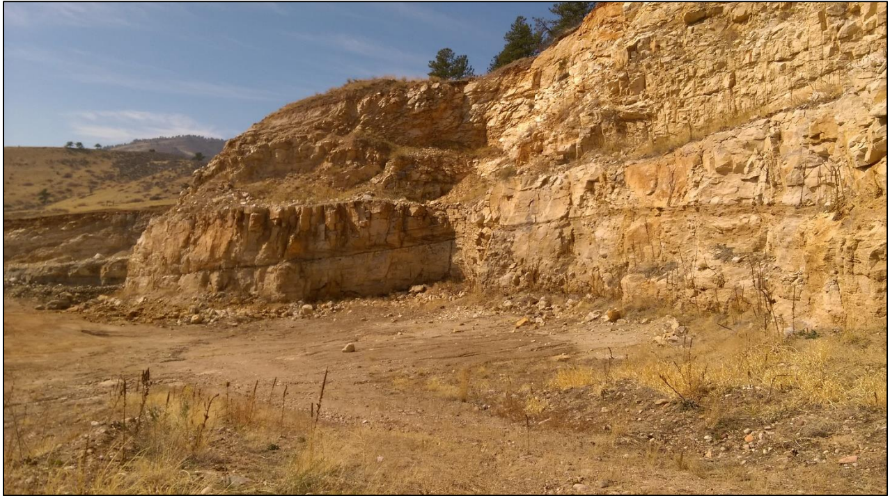
Photo 3. View looking southwest from pit floor, showing western highwall. Note highwall bench slopes have gradients of approximately 0.5H:1V.
