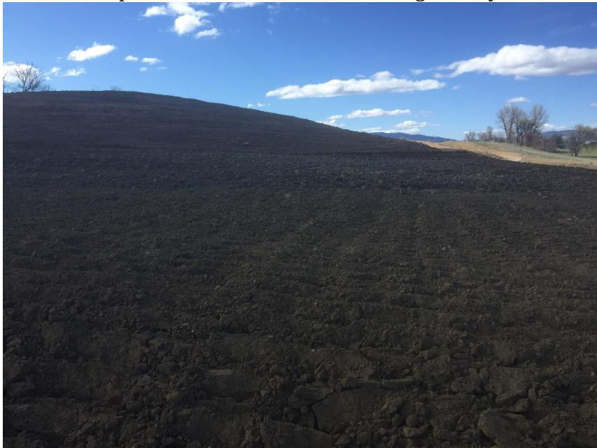
Photo 5 – Topsoil Pile and Disturbed Area
