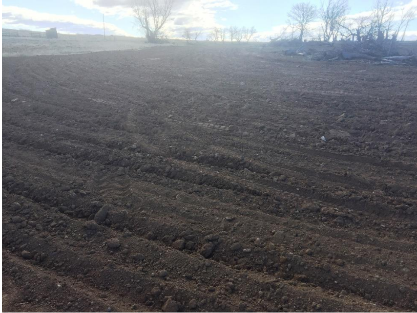
Photo 4 – Topsoil Contoured to AOC Blending in Very Well
