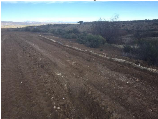
Photo 3-Wattles Along Reclaimed North Ditch
