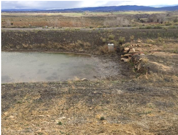
Photo 1 – Pond 001 Discharge Structure
