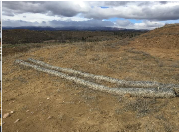
Photo 6 – Ring Ditch with Sediment Trap
