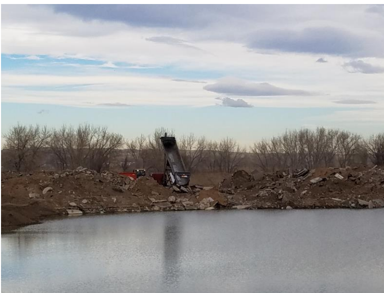
Figure 2. Concrete/dirt being backfilled into the pit.
