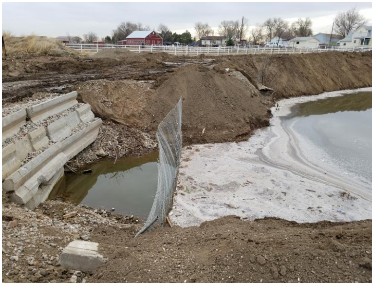
Figure 4. Pit outlet to the South Platte River, northwest end of the pond.
