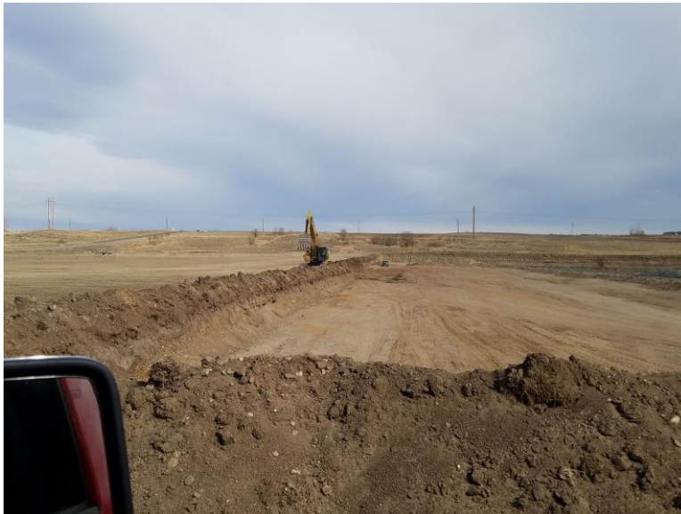
Figure 4. CEC stripping OB in advance of the pit.
