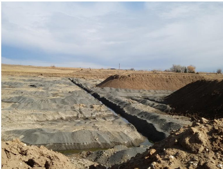
Figure 2. The south central pit area looking north.
