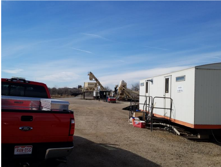
Figure 1. HMA Plant from the scalehouse looking south
