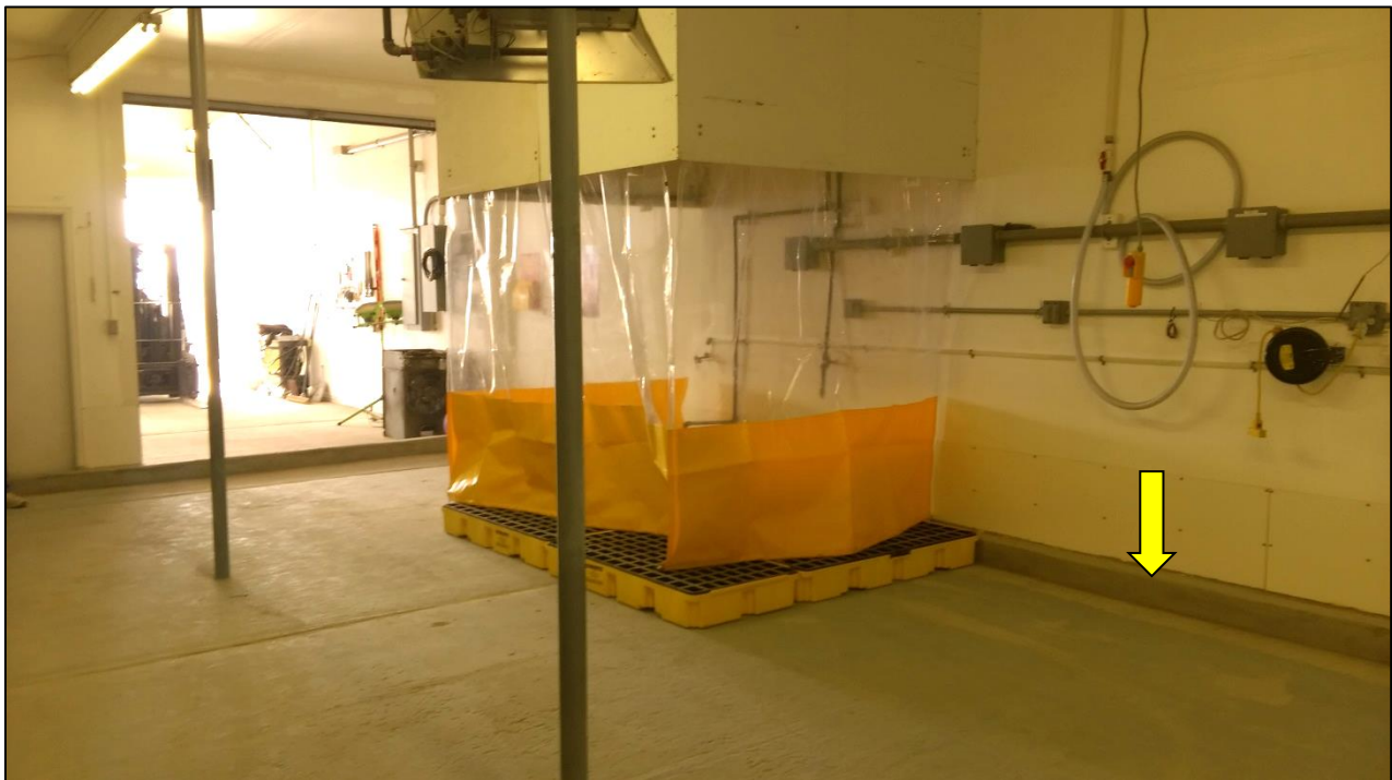
Photo 2. View of "wet lab" where designated chemicals would be used and stored during proposed milling process. Note concrete curb wall constructed around perimeter of room (indicated with arrow).
