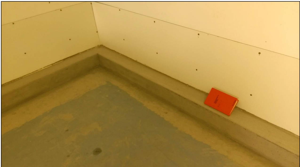
Photo 6. Close-up view of 5 inch high concrete curb wall that was constructed around perimeter of "wet lab". Orange 7-1/2 inch long field book for scale.
