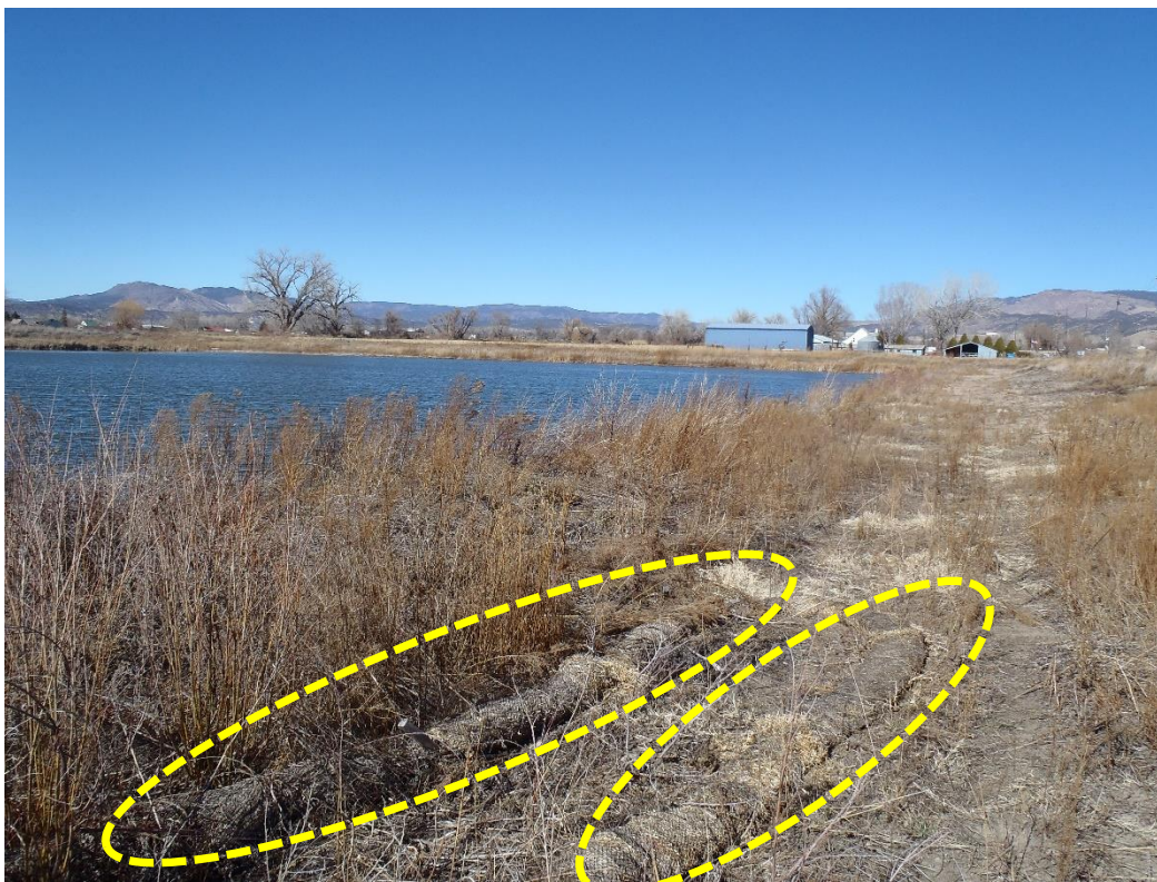
Photo 3. Straw wattles were observed on the east side of the west parcel.
