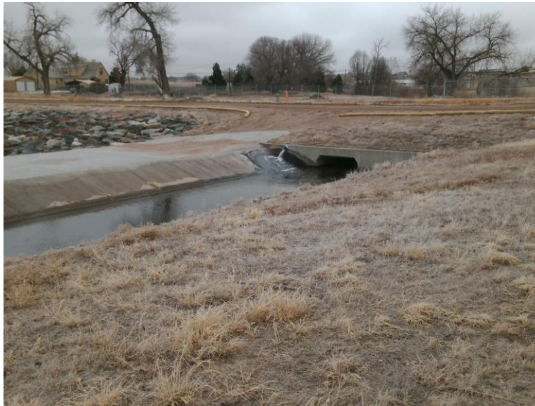
Figure 1. Water discharging from mounding drain into the First Creek Channel north of the site office.
