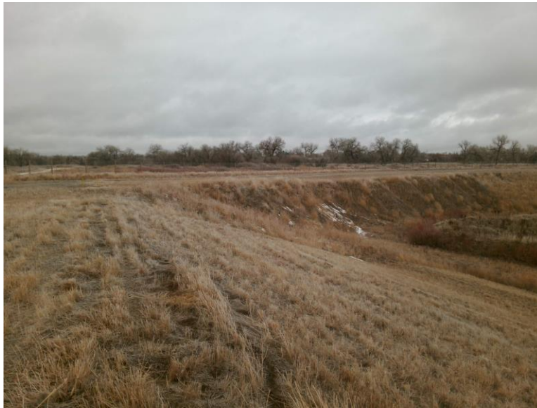
Figure 1. Southwest corner of the Reservoir, steep pit slope that will need to be graded to a 3:1.
