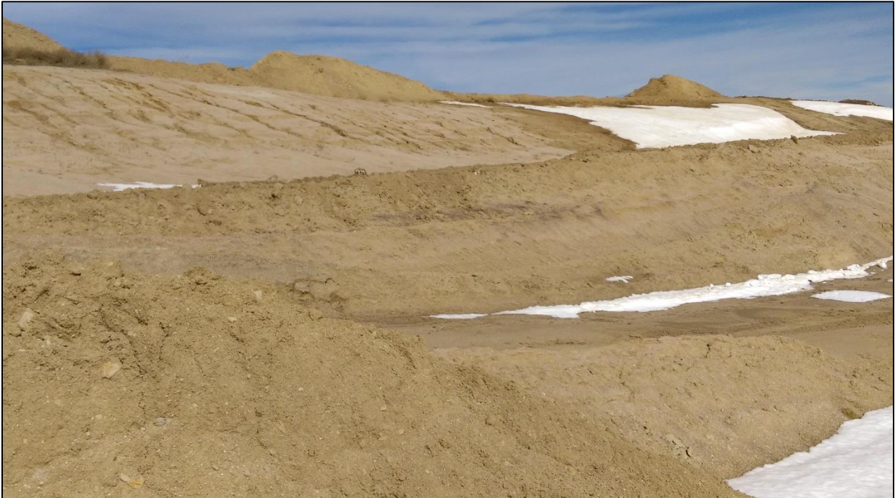
Photo 6. View of eastern portion of northern pit wall, showing slope gradients of approximately 3H:1V. Note presence of erosional rilling along top of slope.
