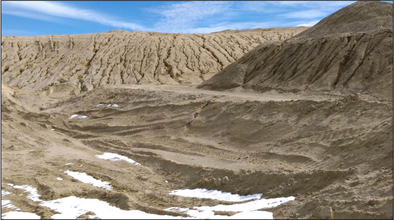
Photo 7. View of northern portion of eastern pit wall, showing slope gradients of approximately 3H:1V. Note presence of erosional rilling and some small gullies forming along top of slope.
