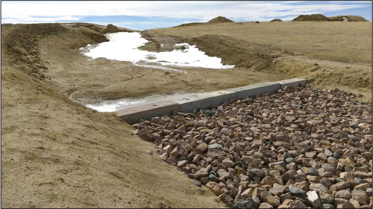
Photo 13. View looking southwest, showing drainage structure constructed at northeastern edge of pit, as approved in TR-4.
