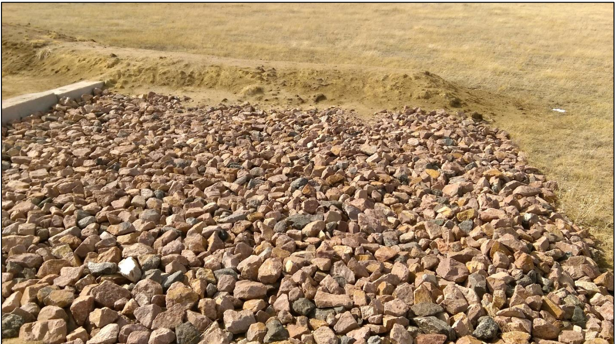
Photo 14. View looking west, showing rip rap portion of drainage structure constructed at northeastern edge of pit, as approved in TR-4.
