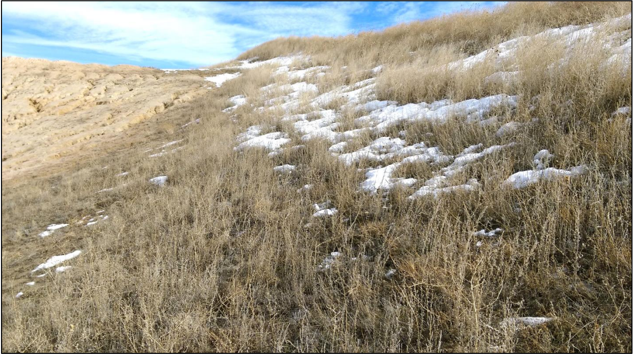
Photo 9. View of eastern portion of reclaimed southern pit wall, showing 3H:1V or flatter slope gradient and established native grasses with some annual weeds.
