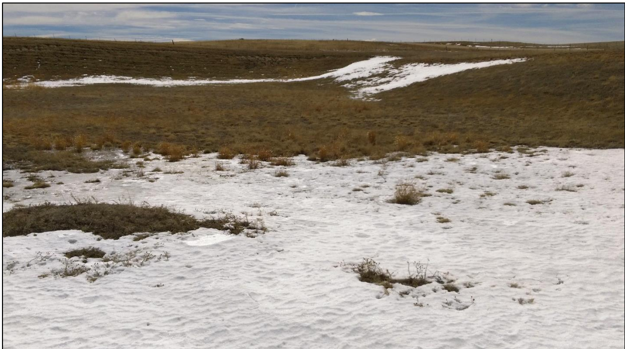
Photo 2. View of western portion of reclaimed area located south of main haul road and west of active pit. Note slopes graded 3H:1V or flatter, and native grasses established across area.
