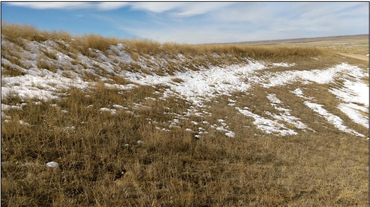
Photo 10. View of western portion of reclaimed southern pit wall, showing 3H:1V or flatter slope gradient and established native grasses with some annual weeds.
