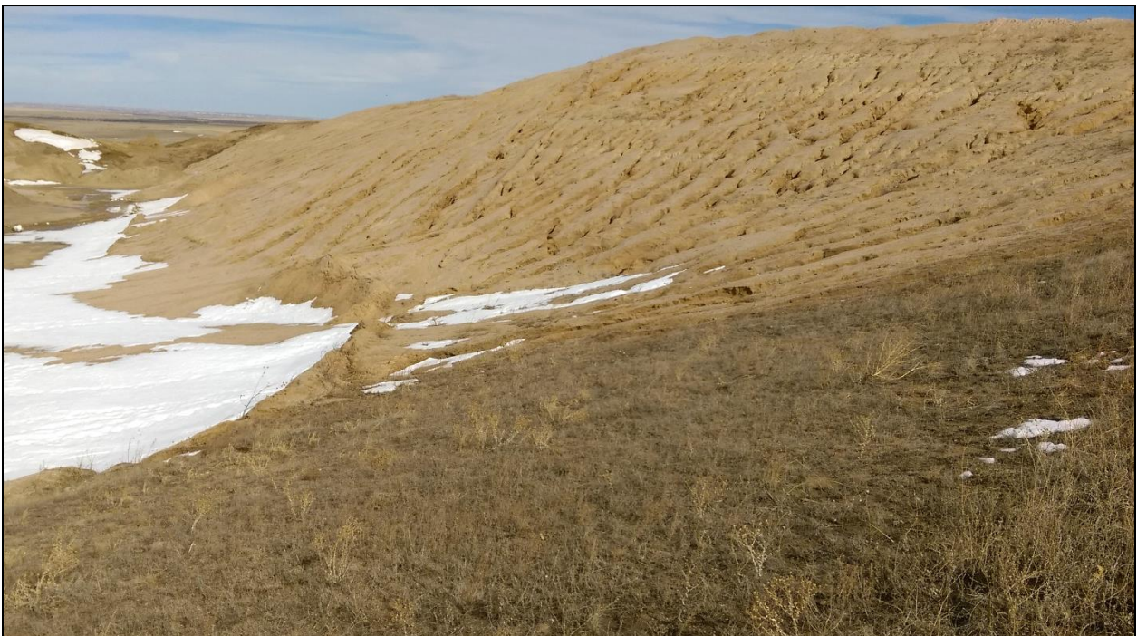
Photo 8. View of southern portion of eastern pit wall, showing slope gradients of approximately 3H:1V. Note presence of erosional rilling along slope. Portion of reclaimed southern wall shown in foreground.
