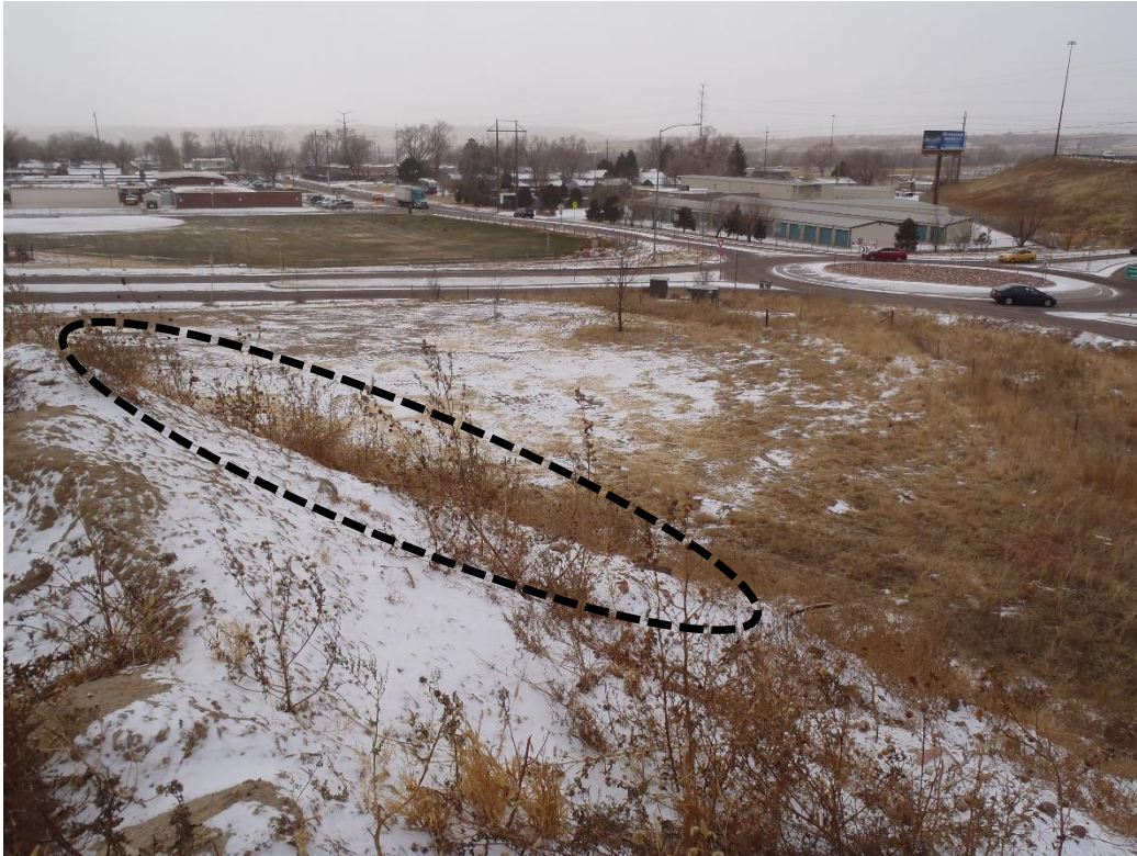
Photo 7. Over steepened southwest embankment slope & newly graded area (looking south from crest).
