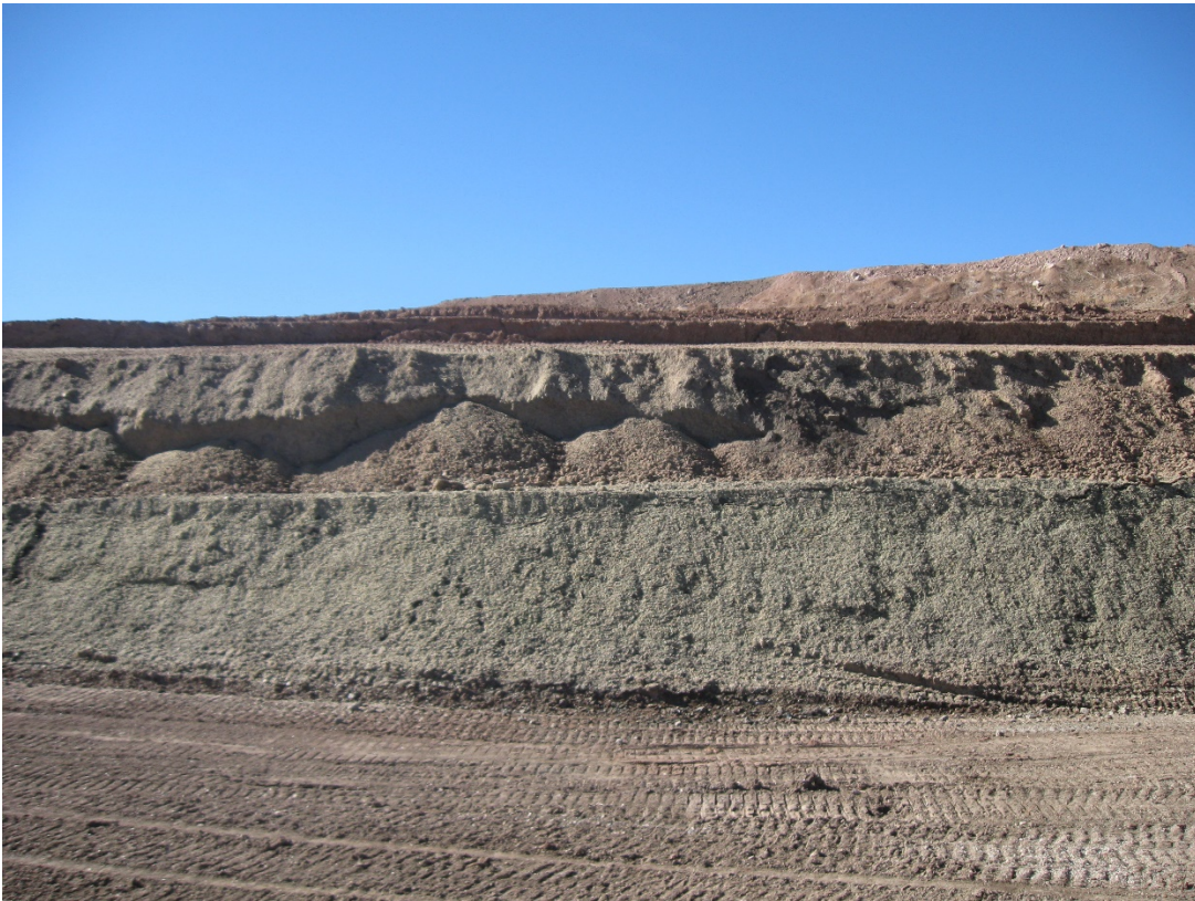
3. Topsoil stockpile stabilization.
