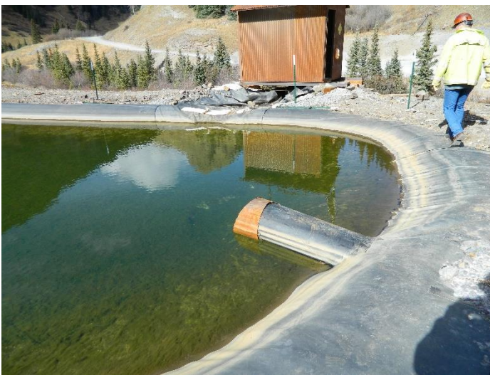
Inlet to treatment from existing discharge collection pond.
