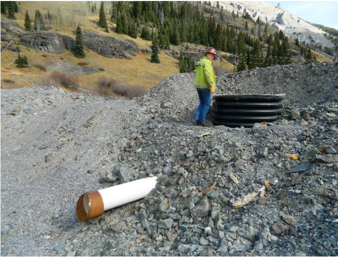
Overflow outlet structure.
