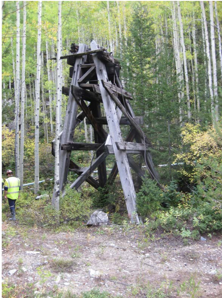
Figure 7: View east of the lower cable tower (Feature 1), 5GN6293.
