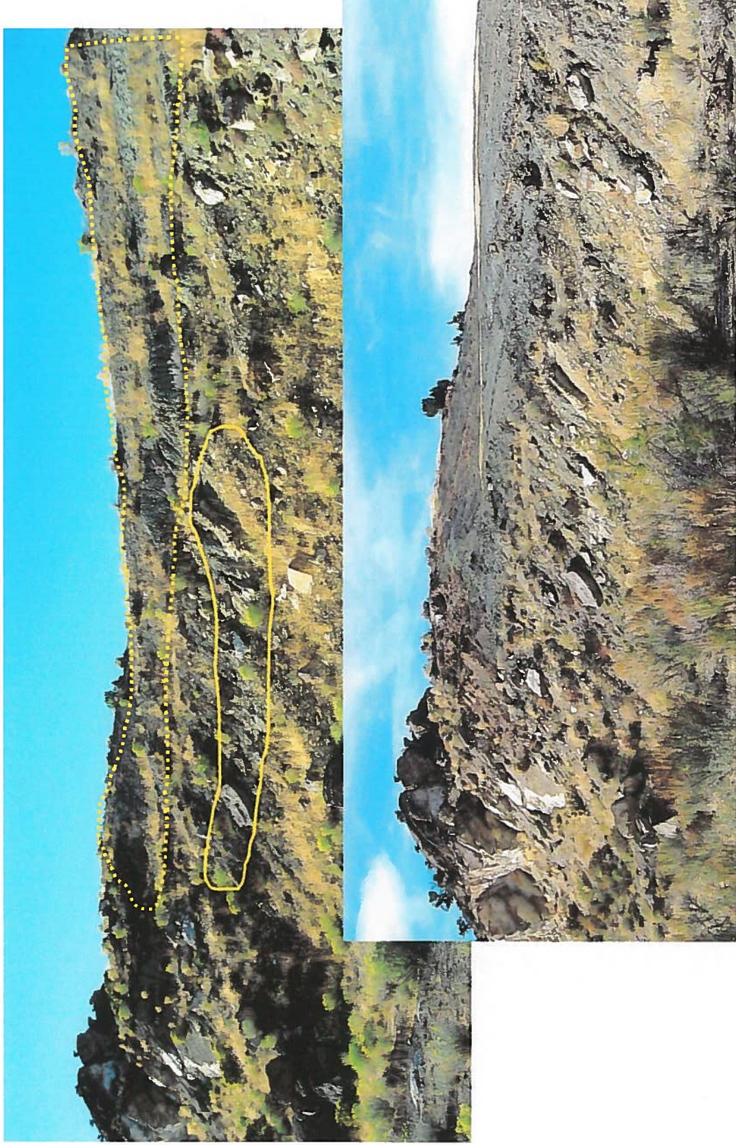
Photo 2 and 3. Bedrock, solid yellow line and the dashed line is the top of the hill that was reduced in height. Lower photo shows hill after contouring.
