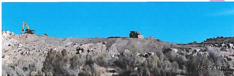
Photo 5. Earthwork in progress.
