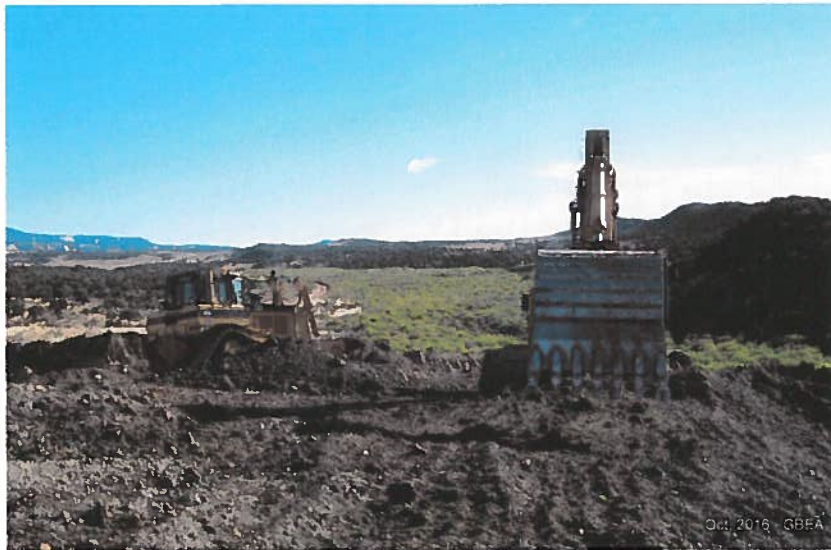
Photo 1. Earthwork in progress (see Photo 11 also).
