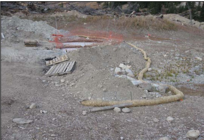
3. Storm water controls at the southern drill pad.
