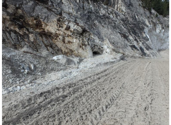
Figure 8: Stormwater directed into utility portal
