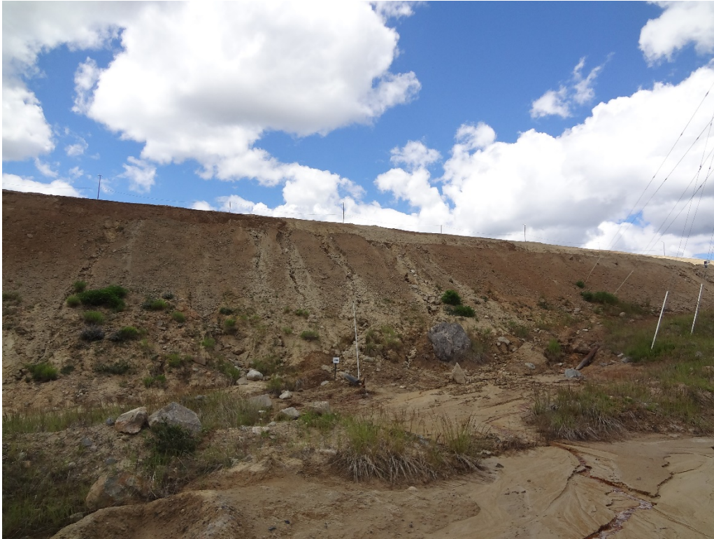
Typ. Horizontal drain in toe of 1-Dam
