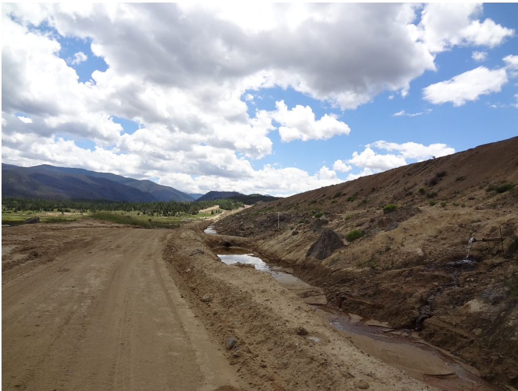
Toe ditch and horizontal drains at toe of 1-Dam
