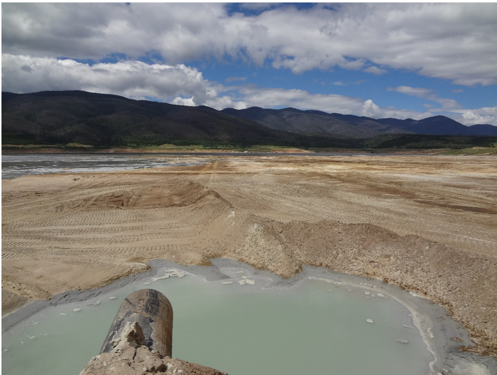
Leadoff between Cells 3 and 4 of 1-Dam looking west
