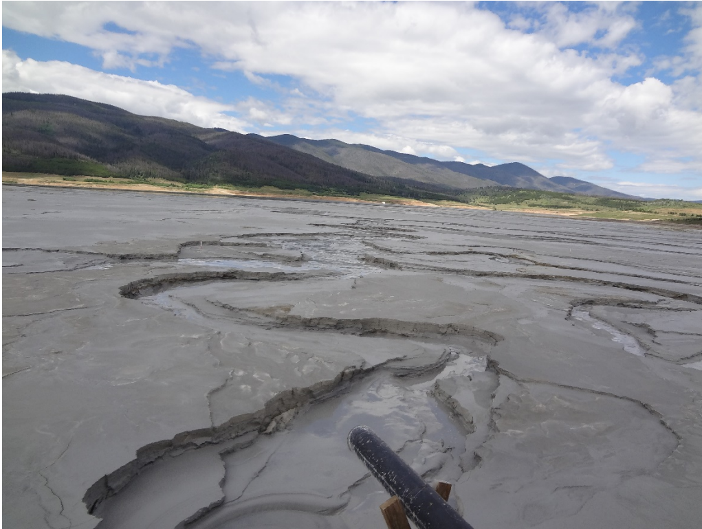
Typical deposition in Cell 2 of 1-Dam
