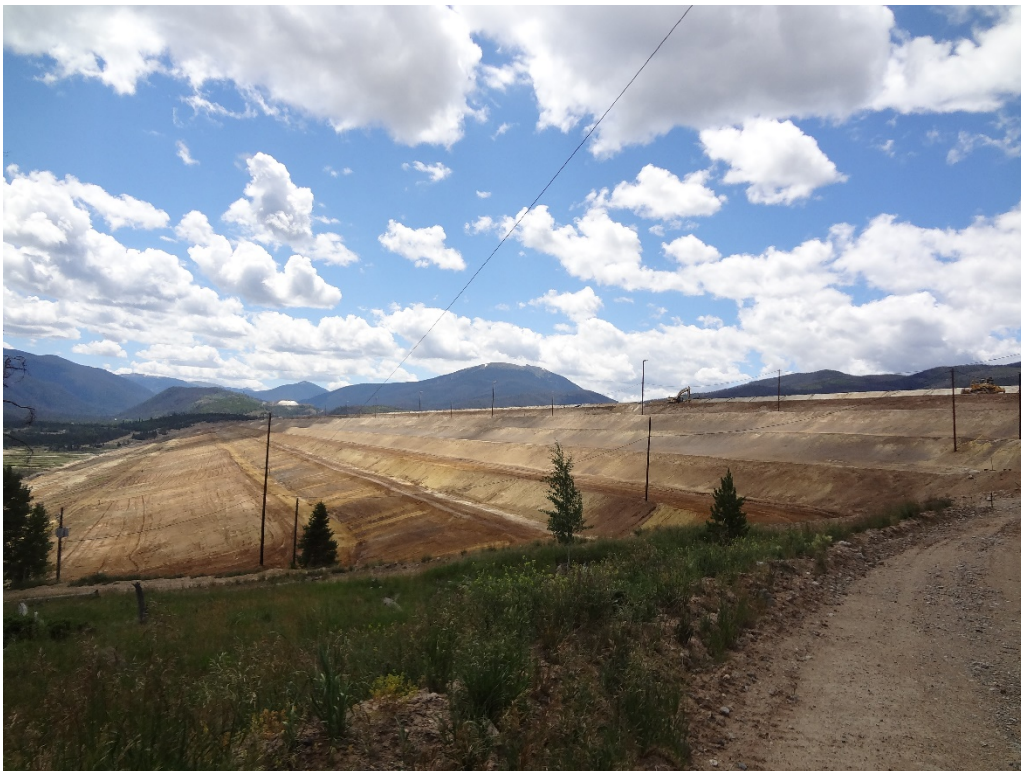
Face of 1-Dam from north end
