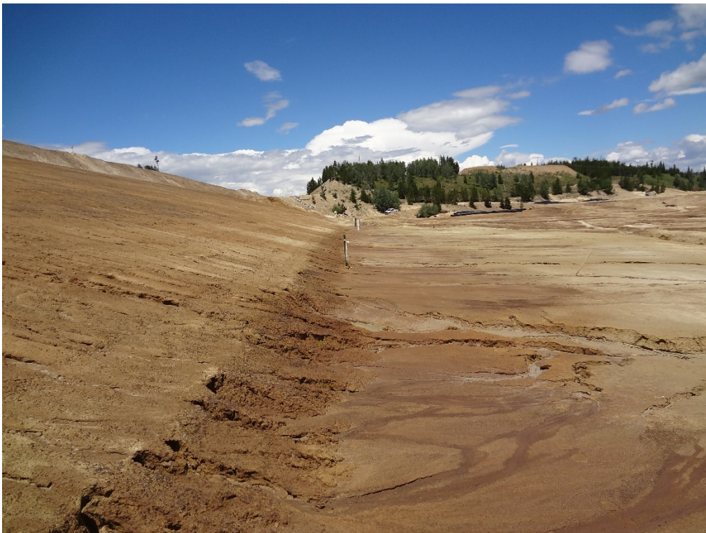
Toe of 3-Dam step looking south at piezometers
