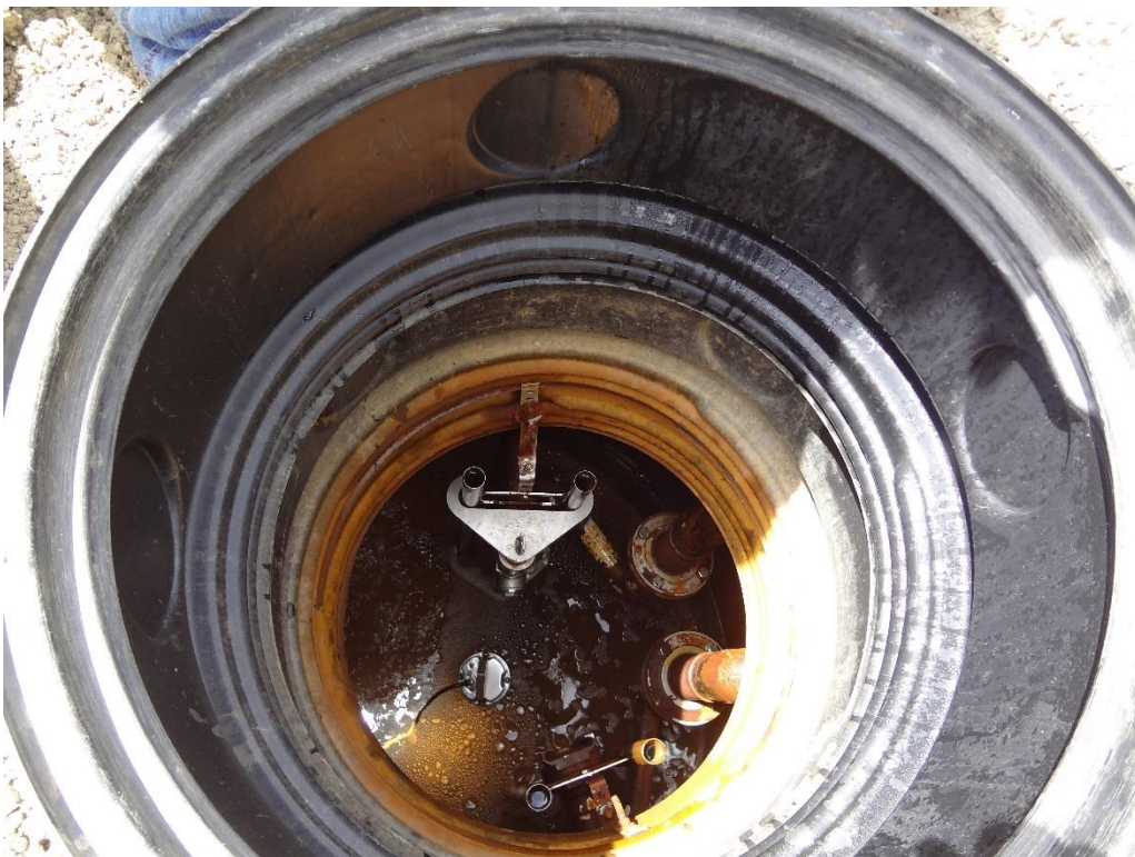
3-Dam Seepage Collection Lower Vault – Replaced Pump
