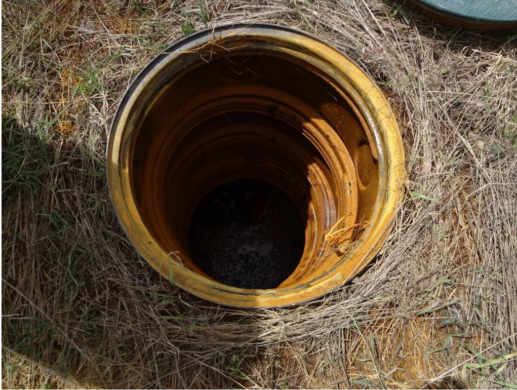
3-Dam Seepage Collection Upper Vault
