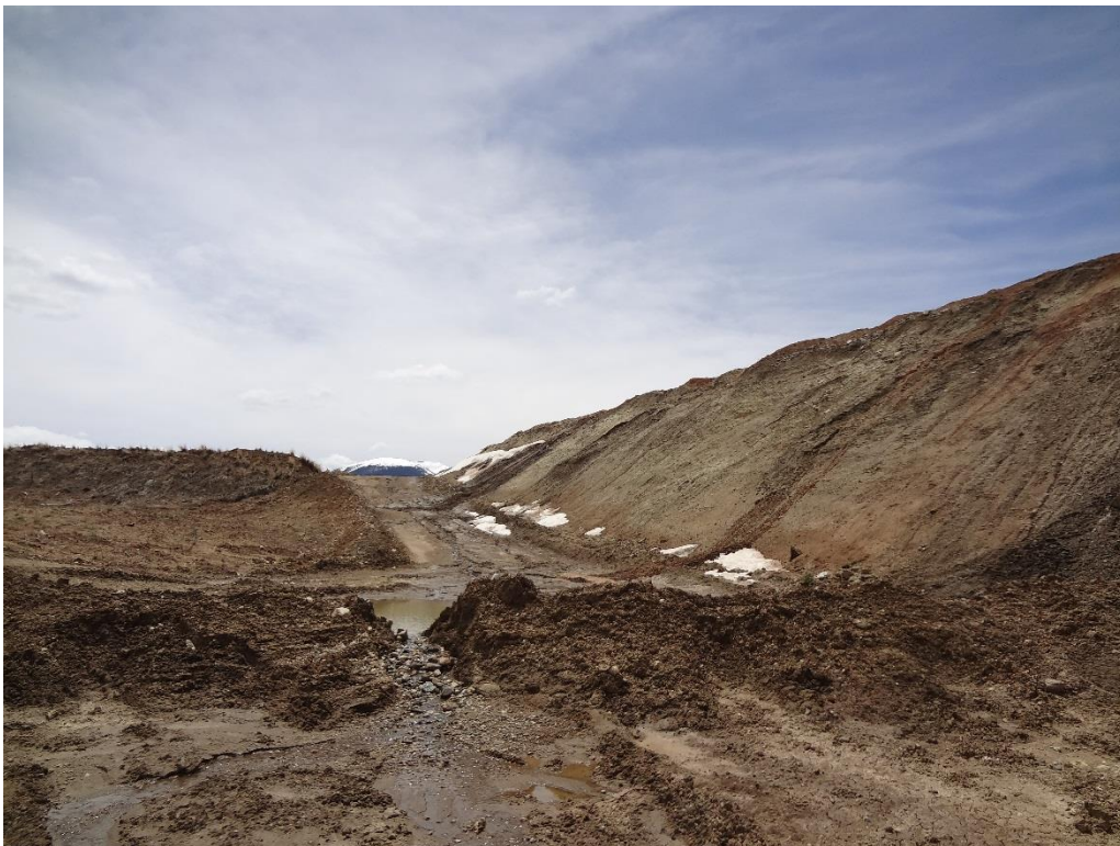
South topsoil stockpile (erosion features)
