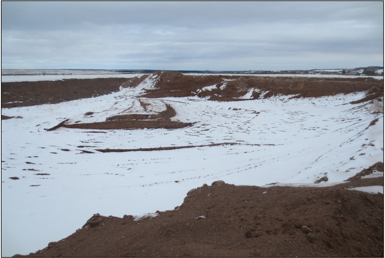
Photo 1: Eastern side of the current exaction. Small highwall along the east side of the pit. The northern side of the pit (left hand side of the photo) has been graded to approximately 2H:1V to 3H:1V.
