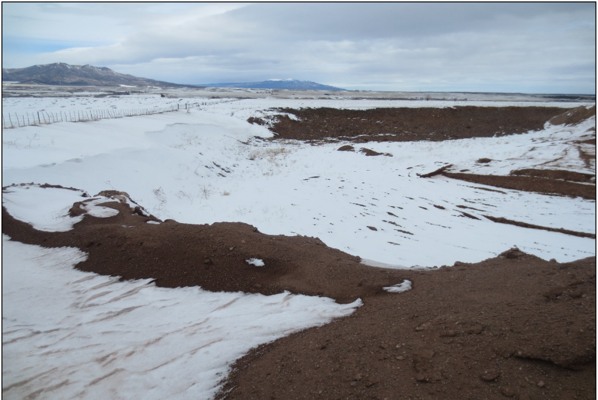
Photo 2: Western side of the current exaction. The northern side of the pit (background) has been graded to approximately 2H:1V to 3H:1V. The western portion of the pit (left hand side of the photo) has been graded to 3H:1V.
