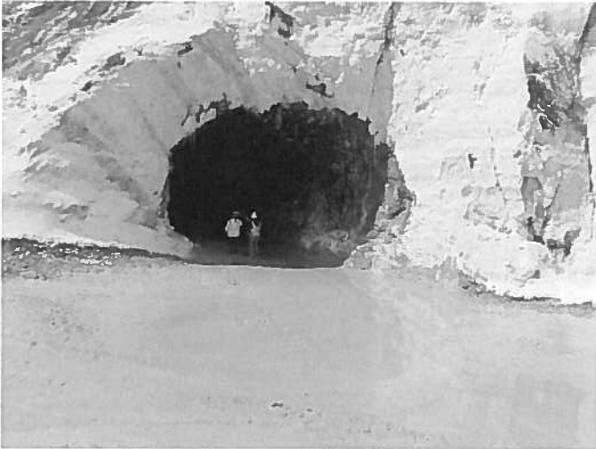
Figure 7: Portal 4 and Washington gallery now utilized for stormwater collection
