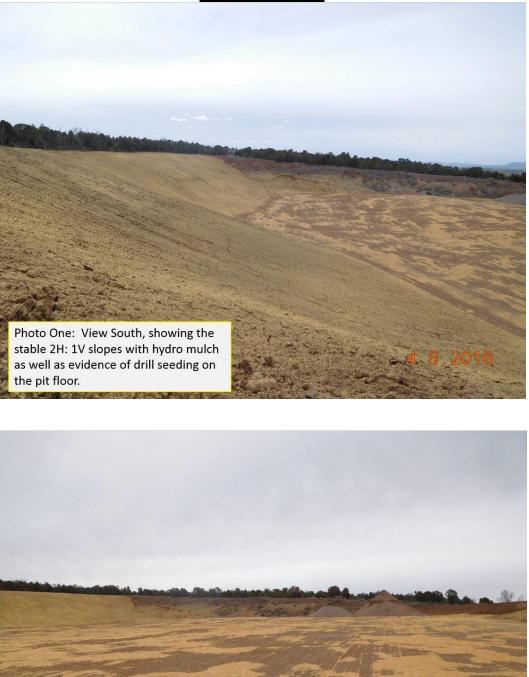
Photo Two: View South, showing the pit floor that has been mulched. Also shown are the stockpiles approved to remain onsite by TR03.
