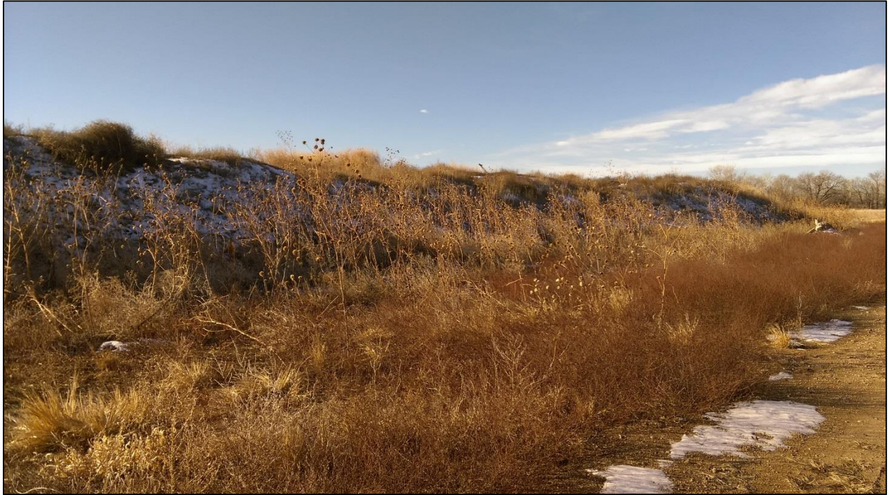
Photo 11. View of northern side of large topsoil berm stored along northern edge of larger excavated pond. Note stockpile is stable with vegetative cover (consisting of grasses and annual weeds).
