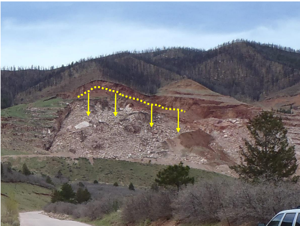
Photo 2. Slide/scarp from current inspection.
