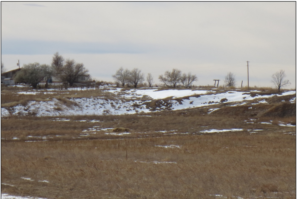
Photograph 2: Southern portion of the pit, this area was mined after the permit was issued. Slopes are approximately 2H:1V, the Operator will need to graded the slopes to 3H:1V or flatter and reseed the entire area.
